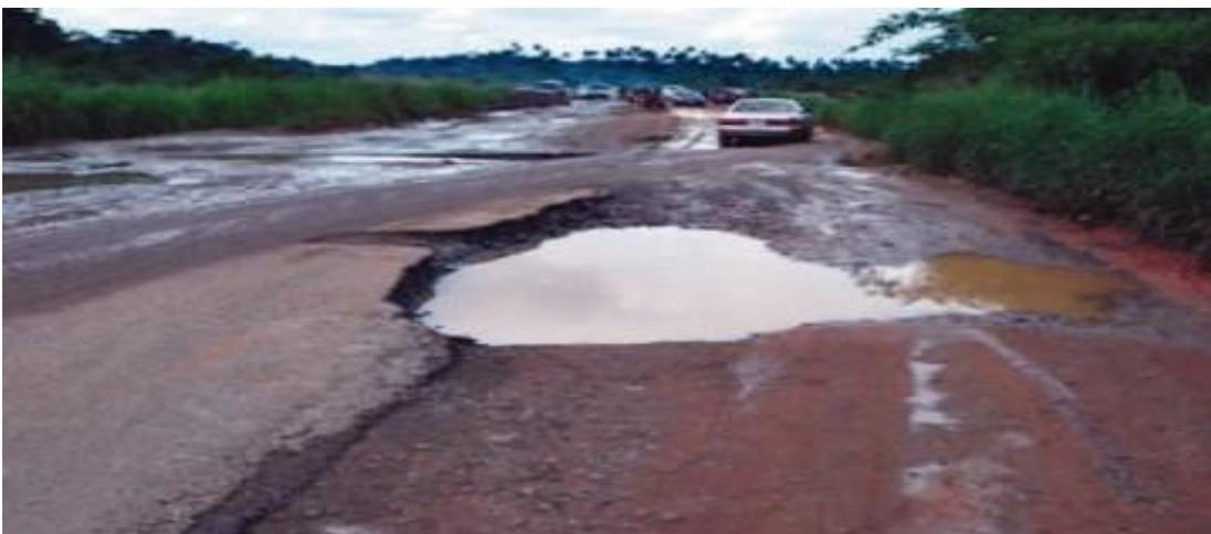
Plate 4: Collapsed portion of Ikorodu – Shagamu road
