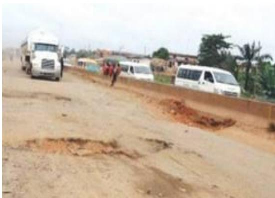
Plate 5: Collapsed portion of Benin - Ore - Shagamu expressway
