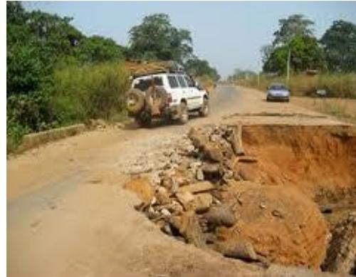
Plate 2: Collapsed portion of Ijebu Ode- Itoikin road
