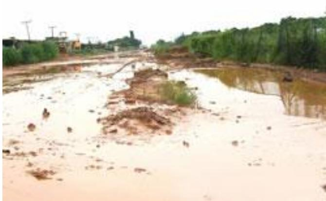
Plate 9: Collapsed portion of Ikorodu - Itoikin - Ijebu Ode road
