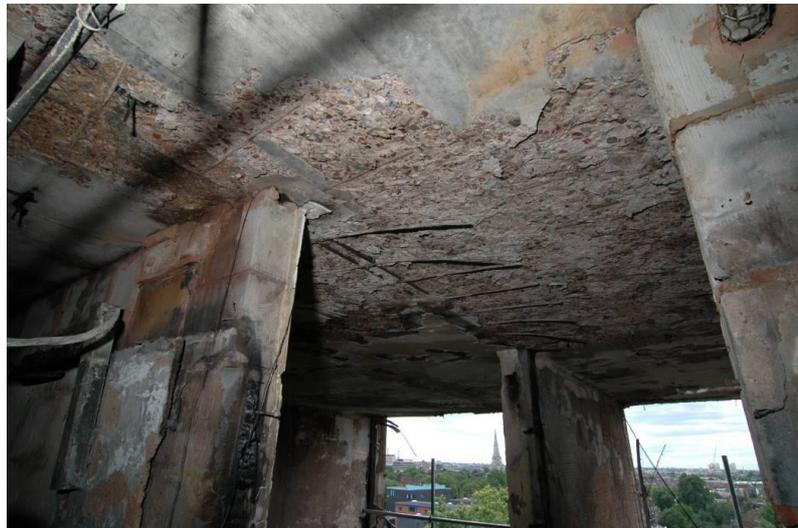
**Figure 64 – Ceiling of Flat 79, lower (11<sup>th</sup>) floor. Note exposure of steel reinforcing bars due to extensive spalling of concrete<sup>140</sup>**
