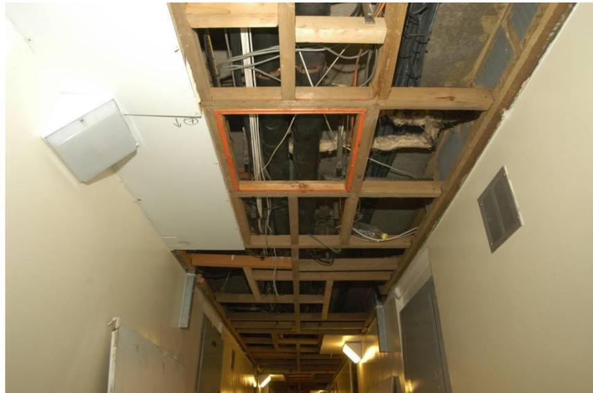
**Figure 65 – Supporting structure of suspended ceiling in the communal corridor of the third floor of Lakanal House. Photograph courtesy of London Fire Brigade (see Appendix**
