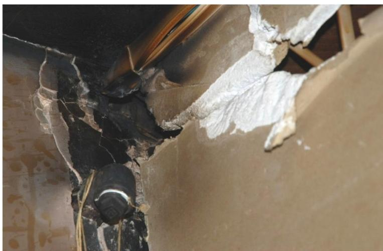
**Figure 55 – Disused pipes passing through wall at location B (DSC\_0010 (cropped) taken by Whitmore LFB photographer, see Appendix C)<sup>140</sup>**
