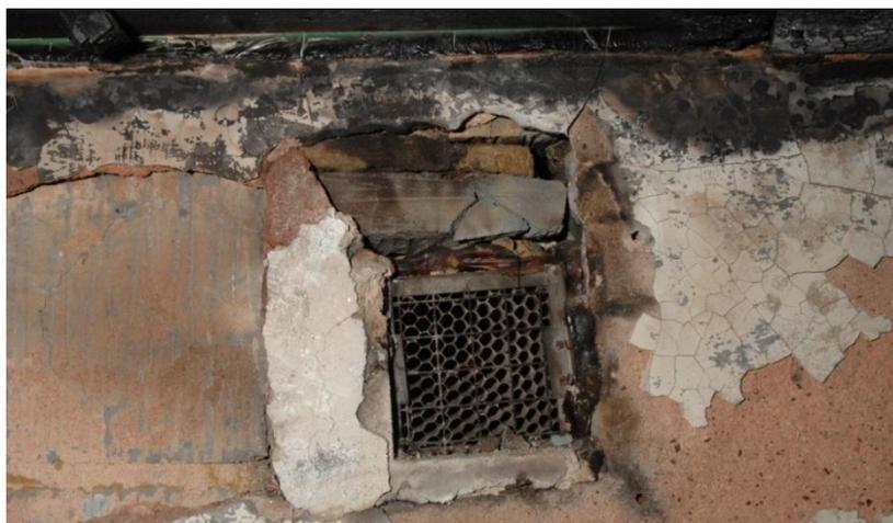
**Figure 57 – Corridor side of filled disused ventilation opening at location C (MPS Photo VF10016, see Appendix B)<sup>140</sup>**
