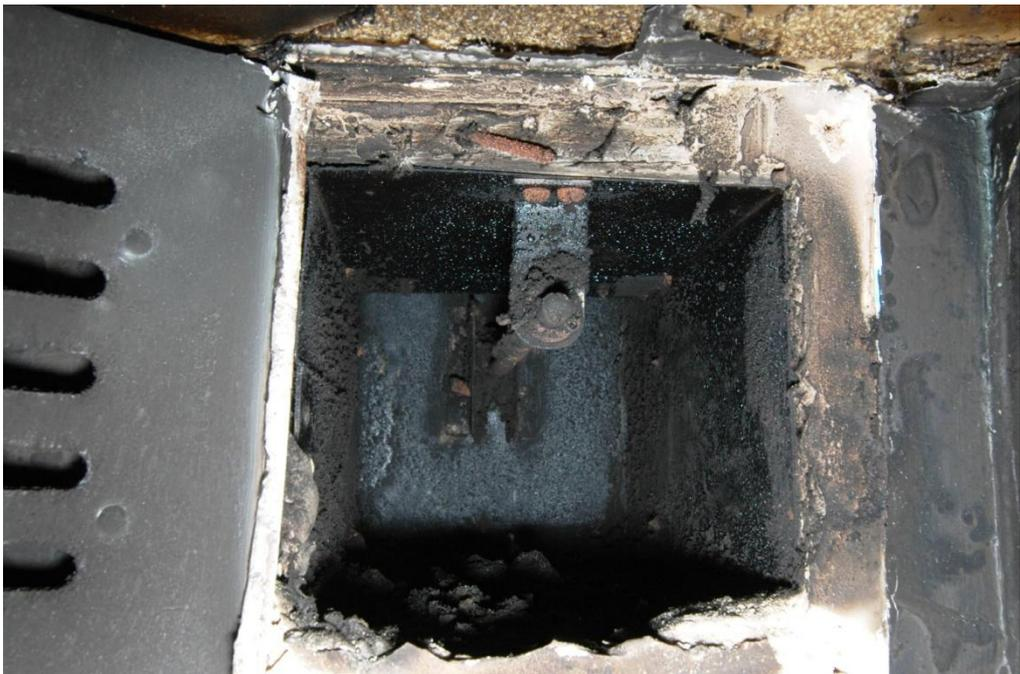
**Figure 131 – Duct and damper behind the grille<sup>140</sup>**
