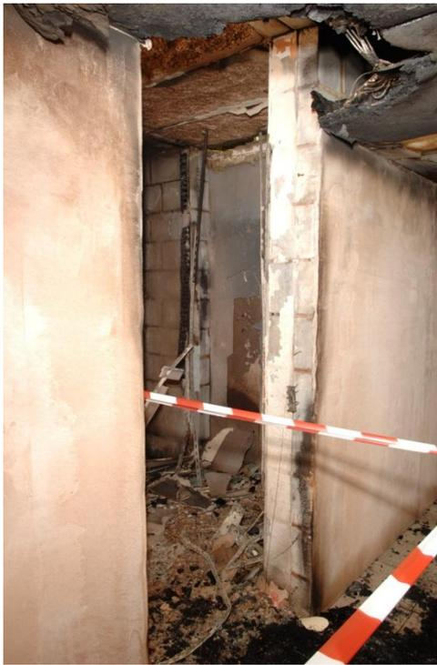
Figure 95 – Space formerly occupied by door D; the flat front door, following the reconstruction fire. Note severe damage to suspended ceiling panels, but no self-sustaining ignition of panels<sup>140</sup>
