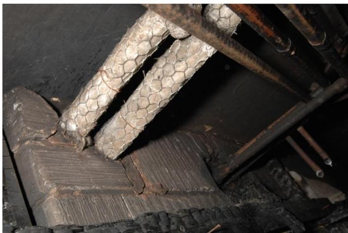
**Figure 60 – Close-up of corridor side of pipe penetration point at location B showing gaps in brickwork above pipe (MPS Photo VF10020, see Appendix B)<sup>140</sup>**
