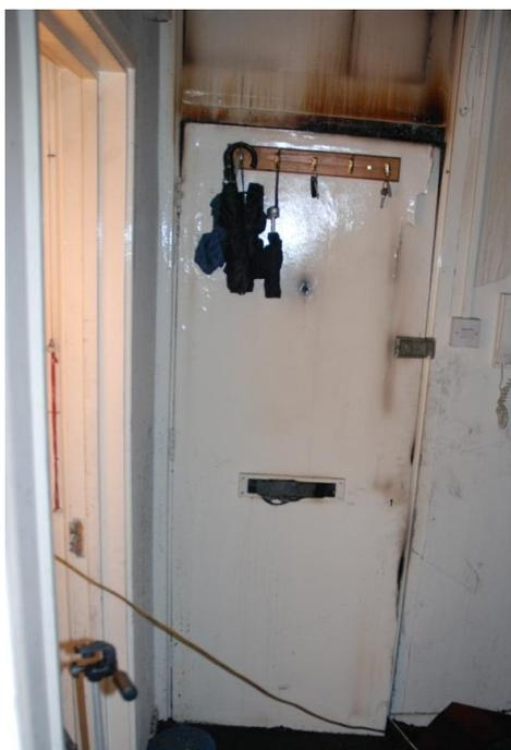
**Figure 134 – Front door of Flat 81, showing discontinuity of damage between top of door and frame plus lack of damage around letterbox and spy hole<sup>140</sup>**
