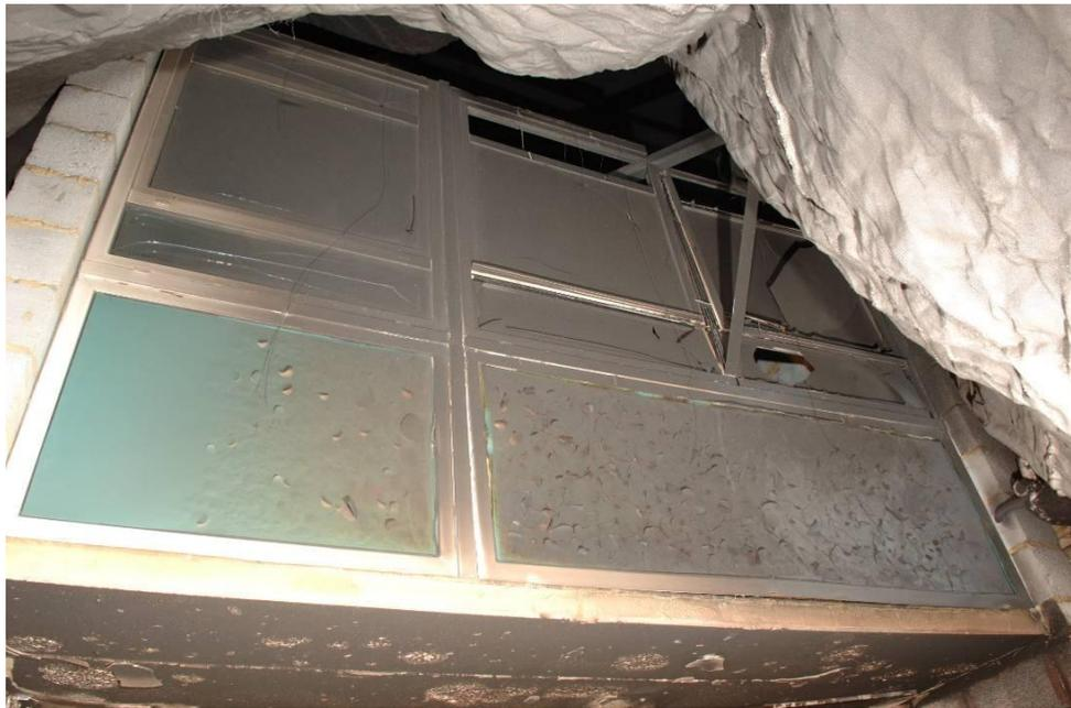
**Figure 91 – Upper floor window set showing damage to glazing plus scorching and distortion of window panels. Photograph courtesy of MPS (see Appendix B) <sup>140</sup>**
