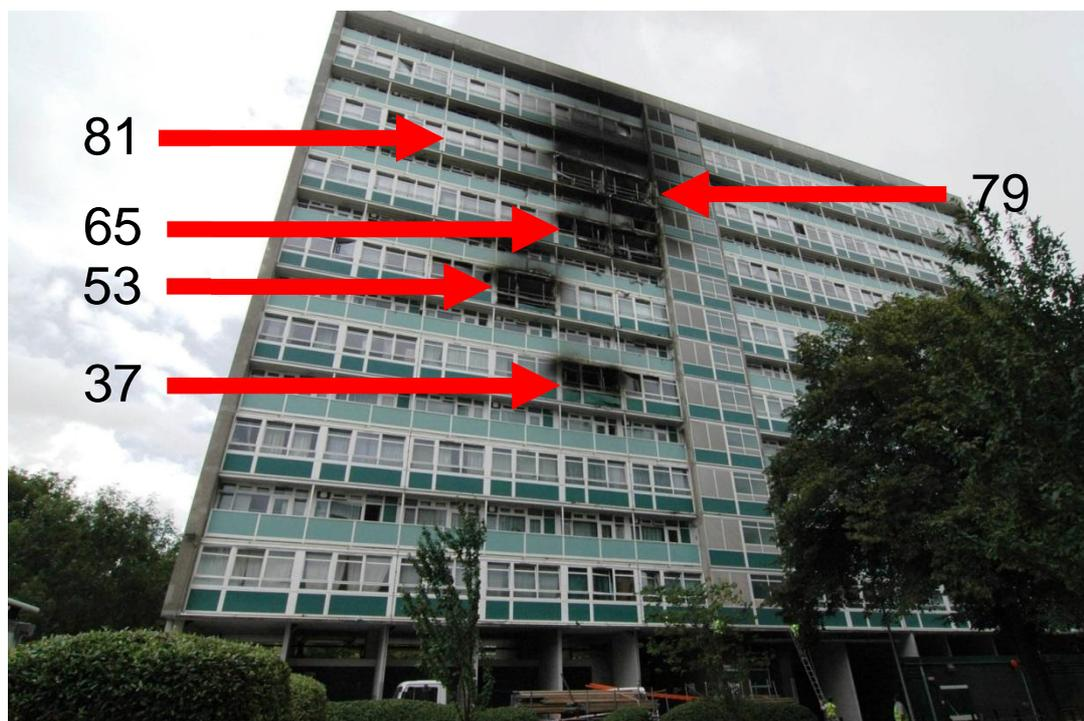
**Figure 50 – West face of Lakanal, showing locations of flats involved in the fire<sup>140</sup>**
