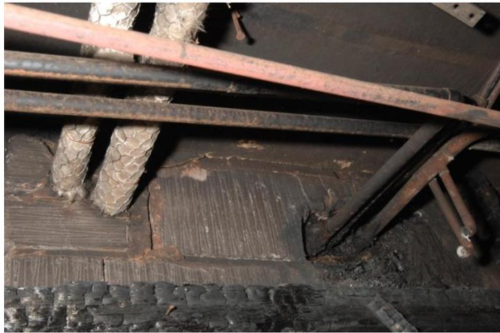
**Figure 58 – Corridor side of pipe penetration points at locations A and B (MPS Photo VF10018, see Appendix B)<sup>140</sup>**
