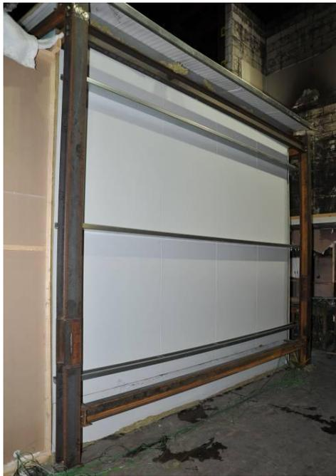
**Figure 143 – External view of steel frame and sandwich panel room prior to reconstruction**
