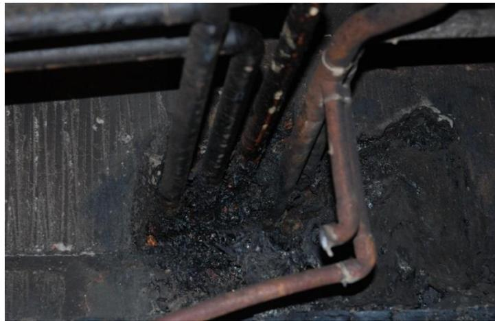
**Figure 59 – Close-up of corridor side of pipe penetration point at location A (DSC\_0114 (cropped) taken by Whitmore LFB photographer, see Appendix C)<sup>140</sup>**
