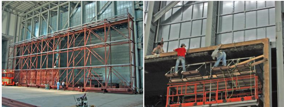
Figure 14. Chamber main door construction and RF gasketting (© 2016 Fleming Steel)
