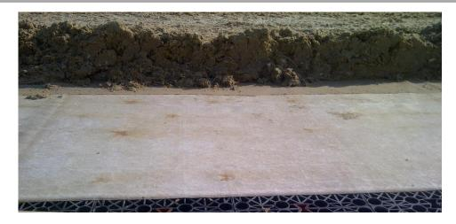
Plate 5.0.2: Synthetic equestrian surface laid to a depth of 150mm over a Permavoid Limited<sup>™</sup> 85 sub-base, separated by a non-woven geotextile membrane.
