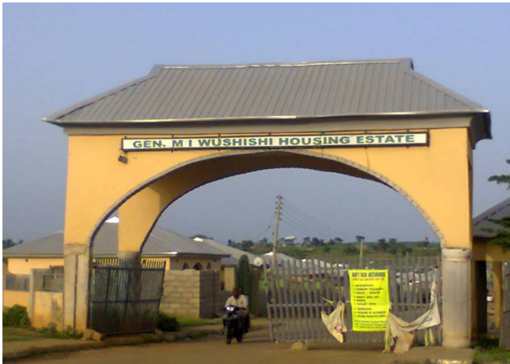
Figure 5.13: The entrance to M I Wushishi Housing Estate Minna - 500 houses
