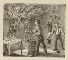
PORTABLE HAND-ENGINE DRILL AND WATER-BUCKET FIRE DRILL.
