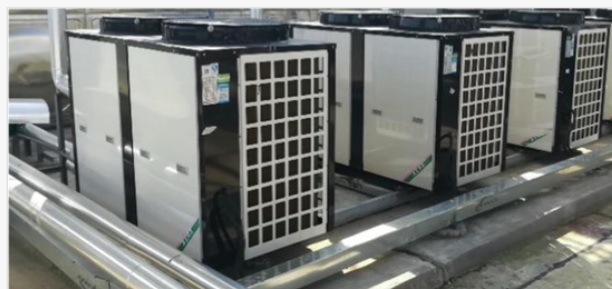
The demonstration project of VI-ASHP installed.
