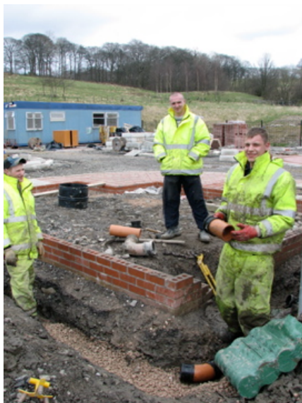
Portable cabin in the distance and three adult trainees learning to dig and lay drains
