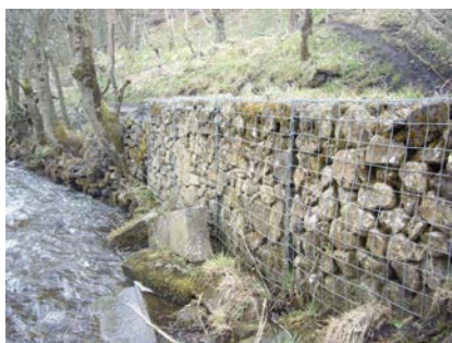
Figure 1.2 reinforced river Roch tributary
