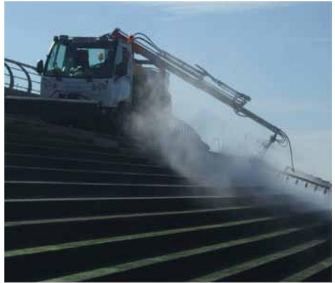
Fig. 2: Power-washing of the precast steps to remove biological growth and minimize slipping hazards
