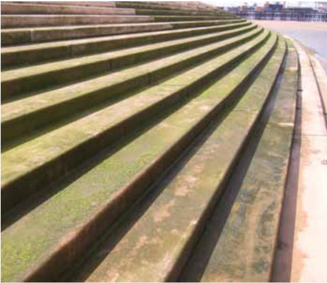
Fig. 1: Precast steps at the Fylde coast of England. The steps have been colonized by algae
