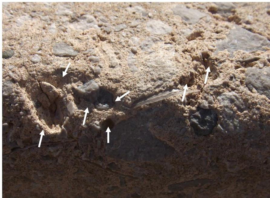
**Figure 8.10** Recently cleaned surface of armour with aggregate liberation (arrowed)
