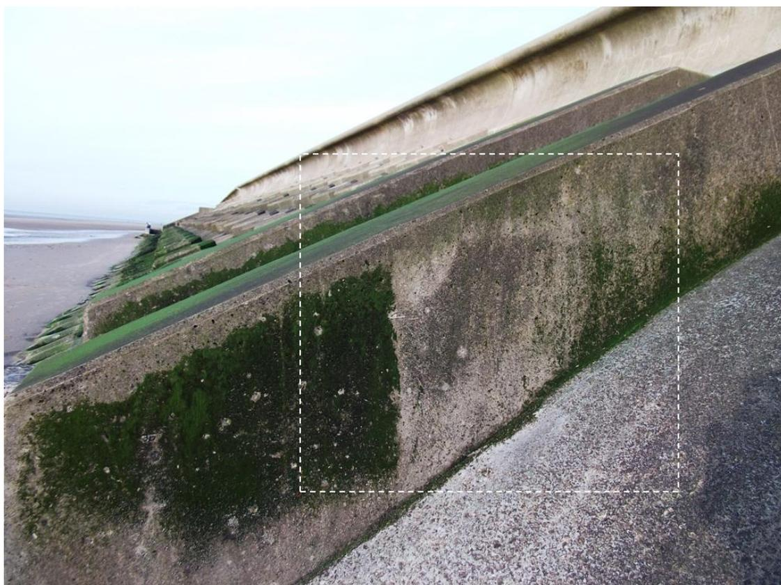
**Figure 6.9**  $\text{TiO}_2$  coated area at study site 1 shows anti-fouling capabilities, image taken April 2011.
