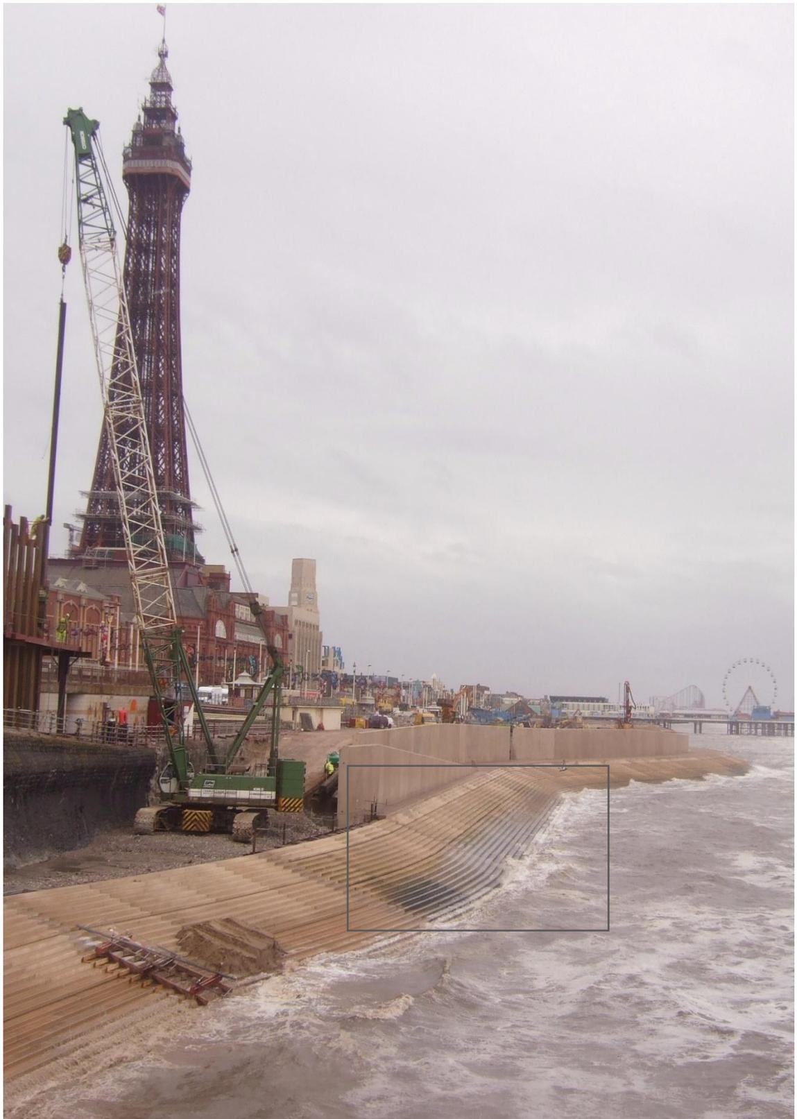
**Figure 1.1** The study site for this research; Blackpool's Central Area Coast Protection Scheme (2010). Recently placed revetment armour units (pH 12 and historically considered not to be bioreceptive at this time) are colonised by *Ulva* (inside rectangle) within weeks.
