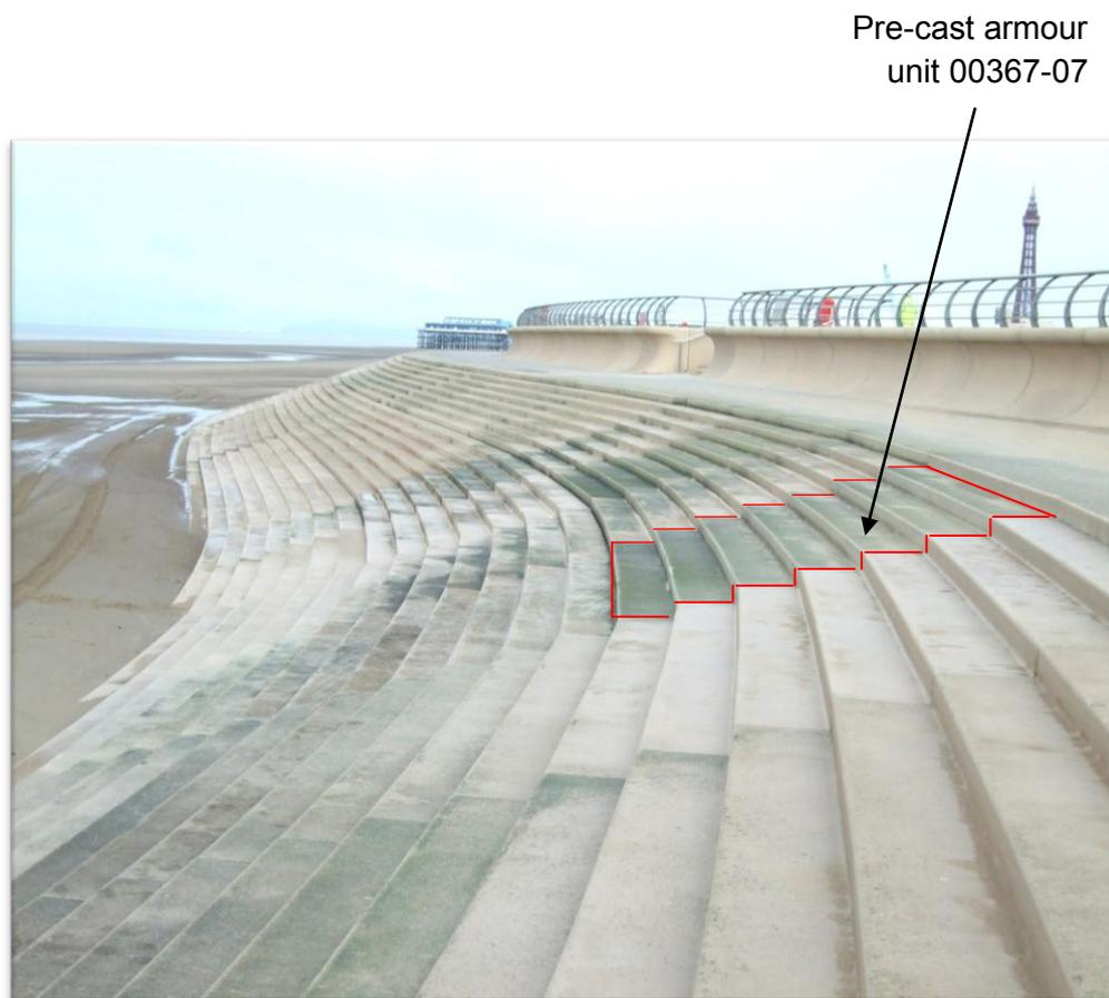
**Figure 3.4** One (of ten studied) of the revetment armour units (arrowed) number 00367-07 set at the study site (Blackpool, north west coast, England) in October 2007.
