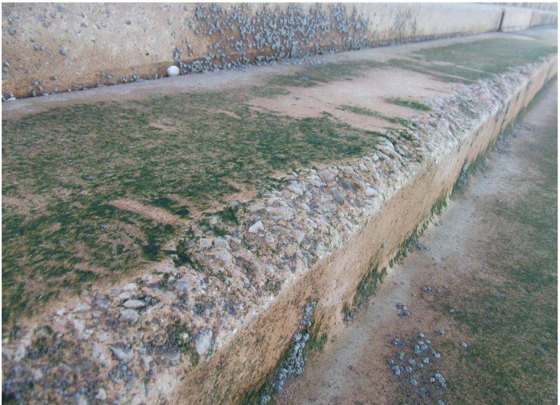
**Figure 4.28** Material loss after five years exposure
