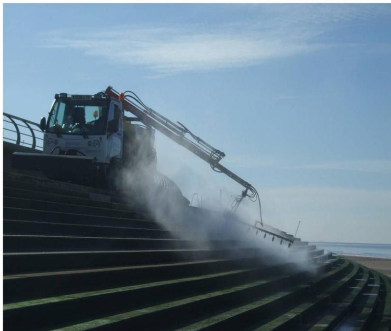
**Figure 3.2** Specially adapted motorised vehicle at the study site, cleaning algae from the revetment armour steps.
