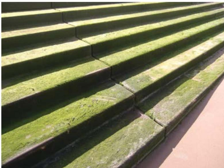
Fig. 2: Revetment armor steps colonized with algae
