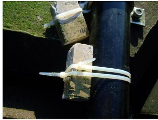
**Figure 6.7** Revetment tiles secured to pipe
