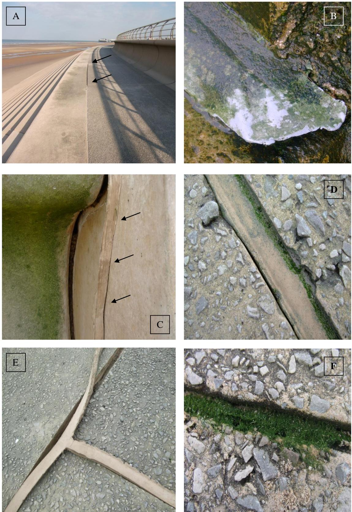
**Figure A5.2** Sealants used at the study site. **A.** Section of sealant missing. **B.** *Ulva* growing on and underneath. **C.** A section of wave wall with sealant fallen away. **D.** *Ulva* at the surface of sealant. **E.** Illustrates a serious trip hazard to the public. **F.** *Ulva* growing under sealant before being removed.
