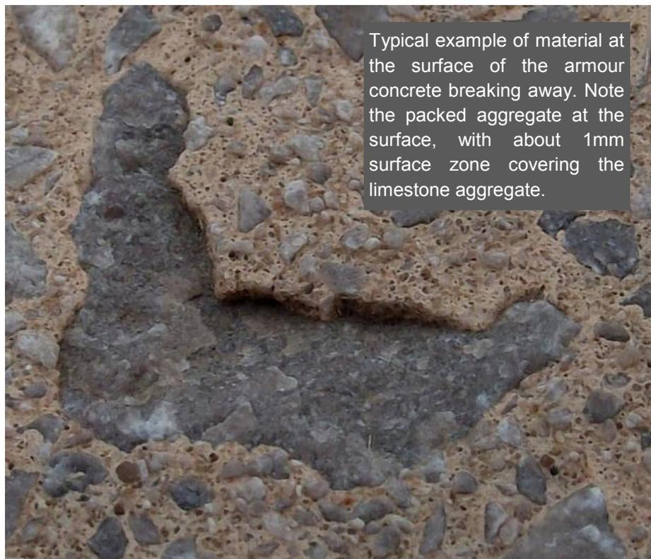
**Figure A3.8** Typical surface zone to revetment armour (after 1 yrs exposure).
