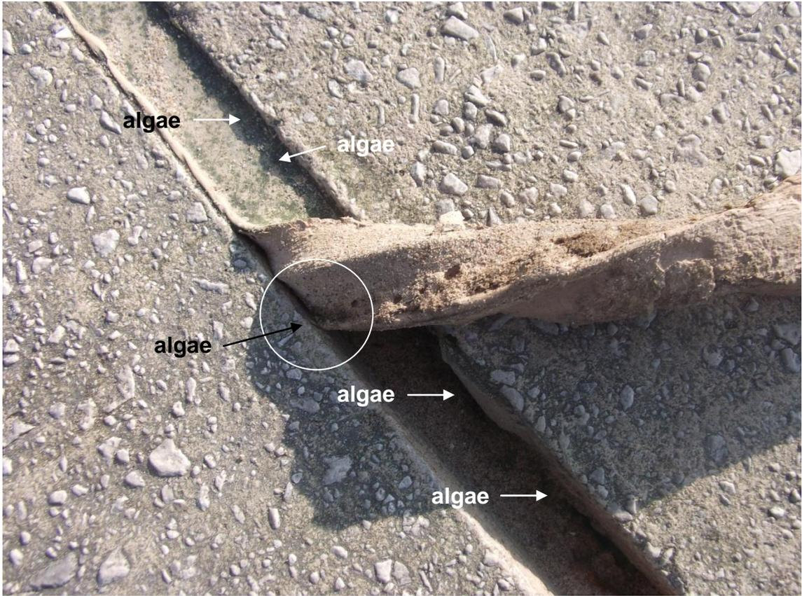
**Figure A5-1** Sealant at the study site. Algae growing under the sealant (arrowed), eventually causing the material to de-bond. Other degradation mechanisms such as cleaning and tidal impact will also play a role.
