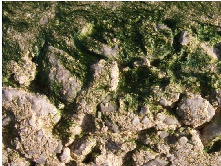
**Figure 8.12** The initial surface has now eroded. Aggregate appearing at the surface of the concrete unit.
