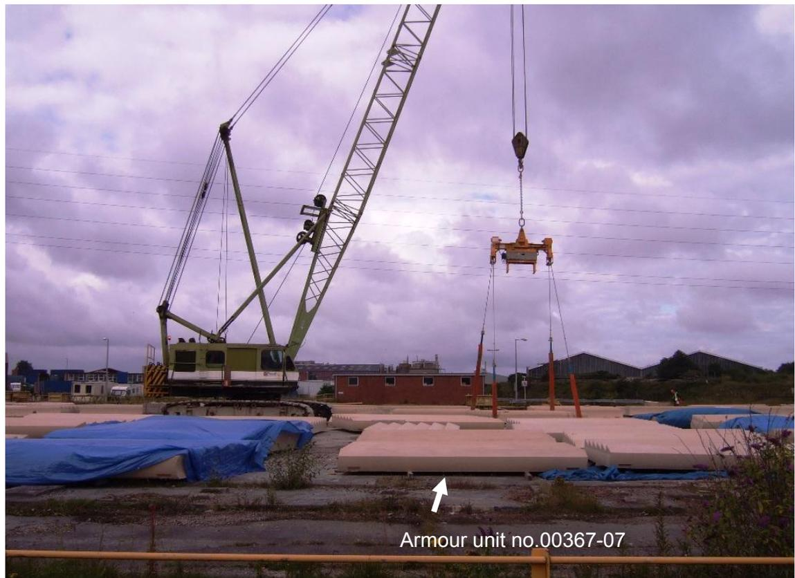
**Figure 3.3** Four point lifting revetment armour at the casting yard. Cast unit number 00367-07 (arrowed) membrane cured, for 28 days at the casting yard (north west England) in 2007.
