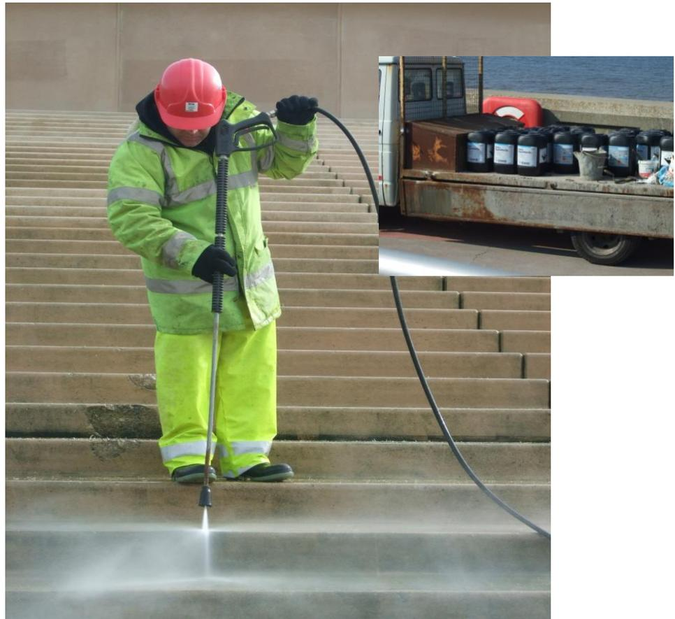
**Figure 3.1** Operative with hand held water jet controlling biofouling with power washing at the study site; inset, dairy hypochlorite (chlorine-based disinfectant) used at the site, video on CD in appendix.
