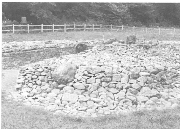
Fig. 14 The restored south-east horn, showing the rounded stones claimed by the excavator as from a former stream bed. Scale in ft. Photograph: RCAHMW (GL3037), Crown copyright reserved
