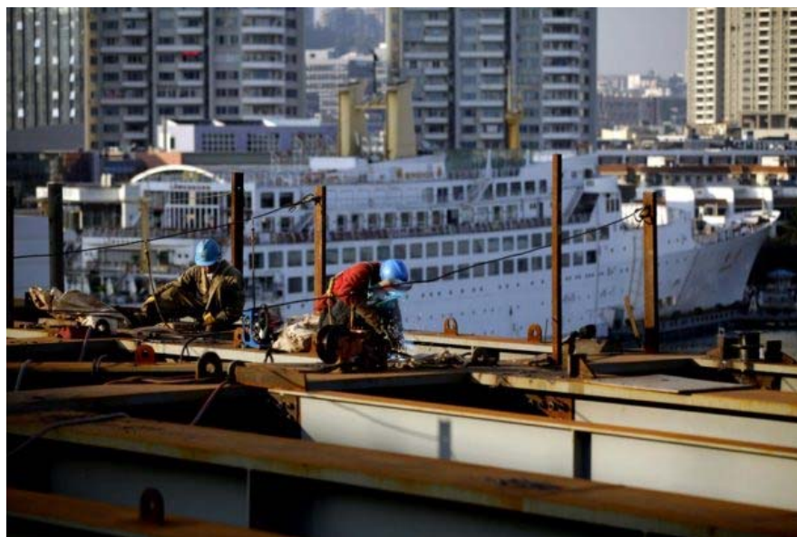
Jan 2016 – Work in progress at the building site (Photo by Design Society)
