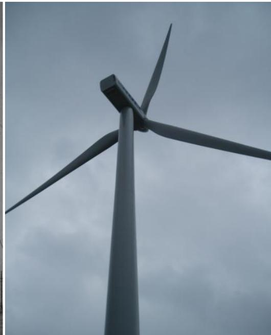
Figure 2-3 Horizontal-axis wind turbine
