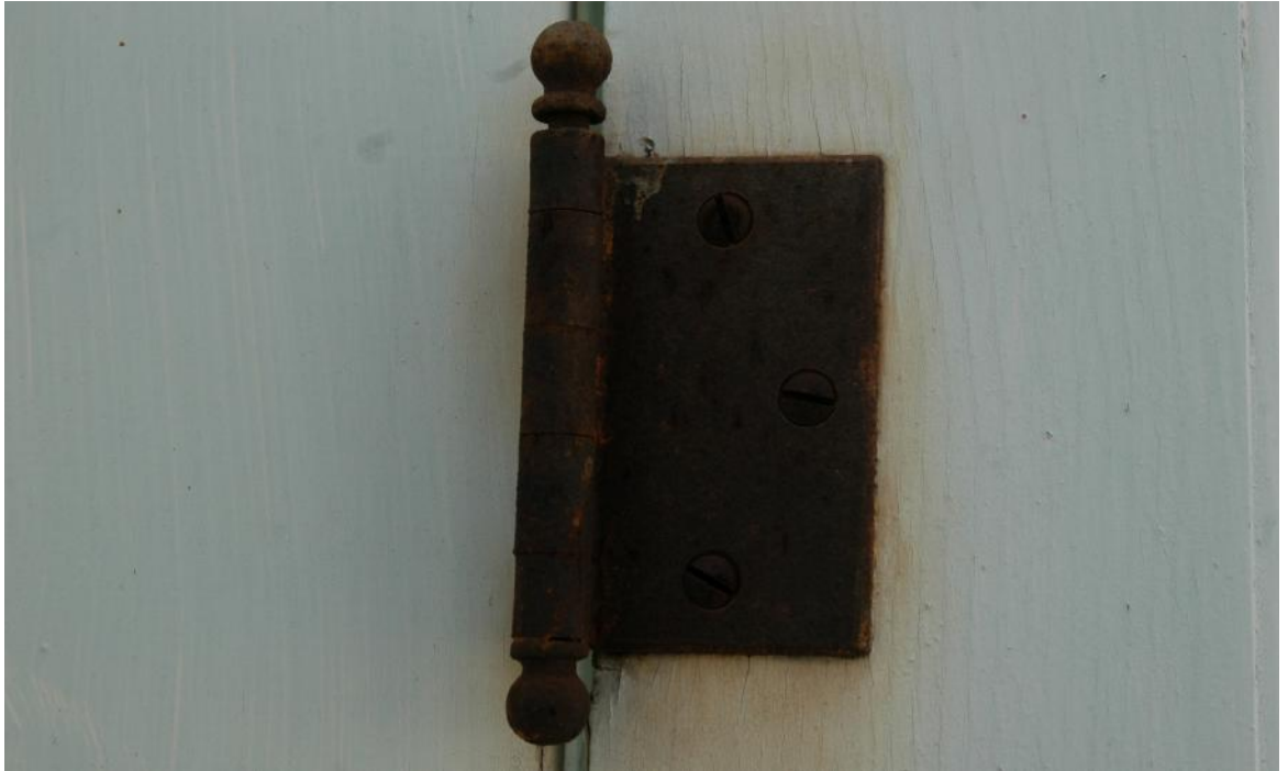
DSC_0442 – Bathroom door hinge hardware.
