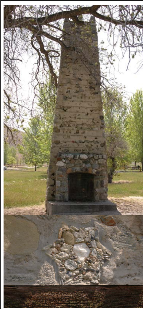
Figure 5.7: Freestanding chimney feature made from native stone. For its location within the complex of Headquarters, see Figure 5.5.
