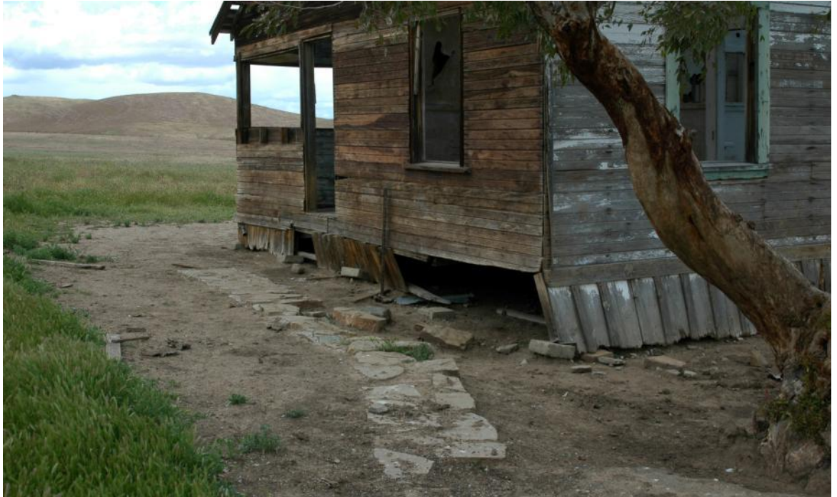
DSC_0298 – View toward west. South end of Dorothy's House with native stone and concrete walk way. Eucalyptus tree to the right of view.
