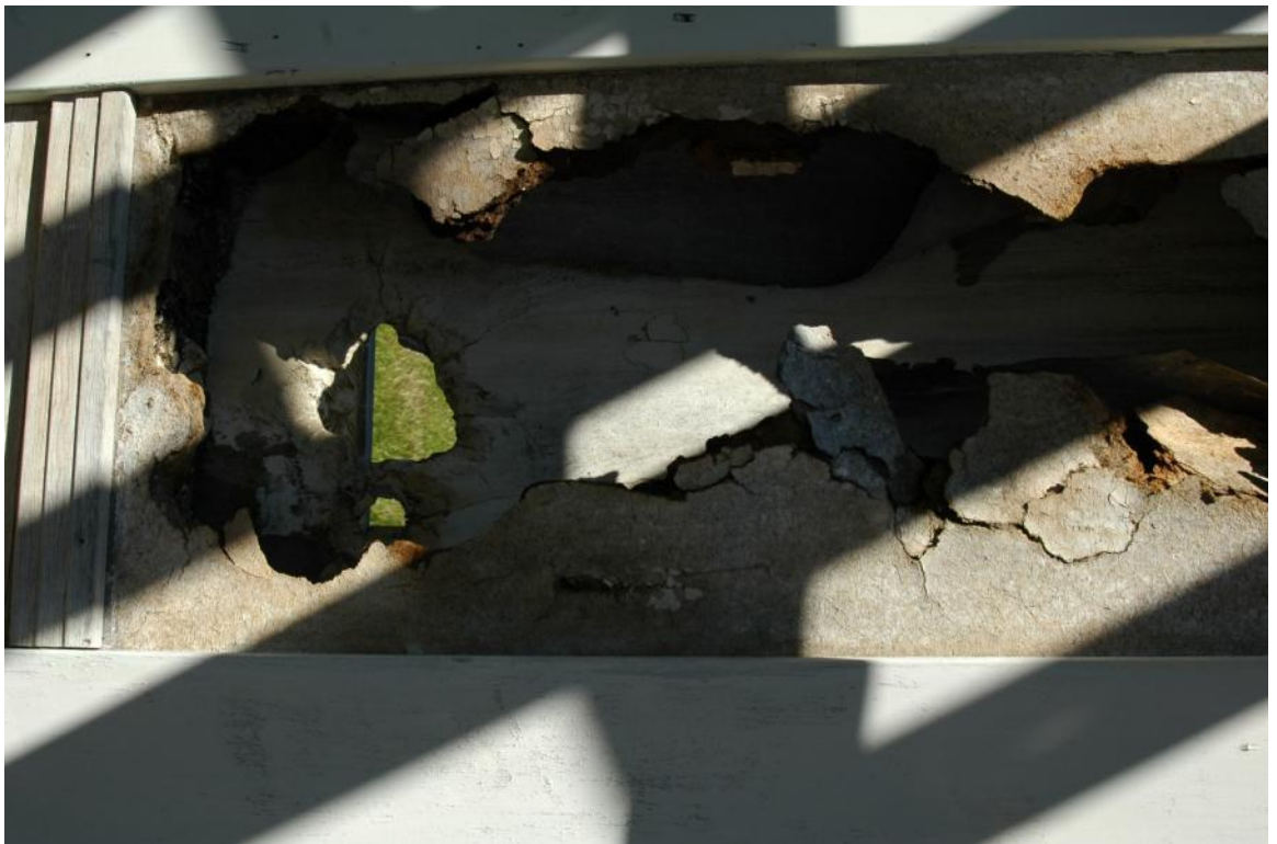
DSC_0445 – View of wall matrix, showing original wood paneling of Dorothy's House, and the sheet rock from when north porch was enclosed.
