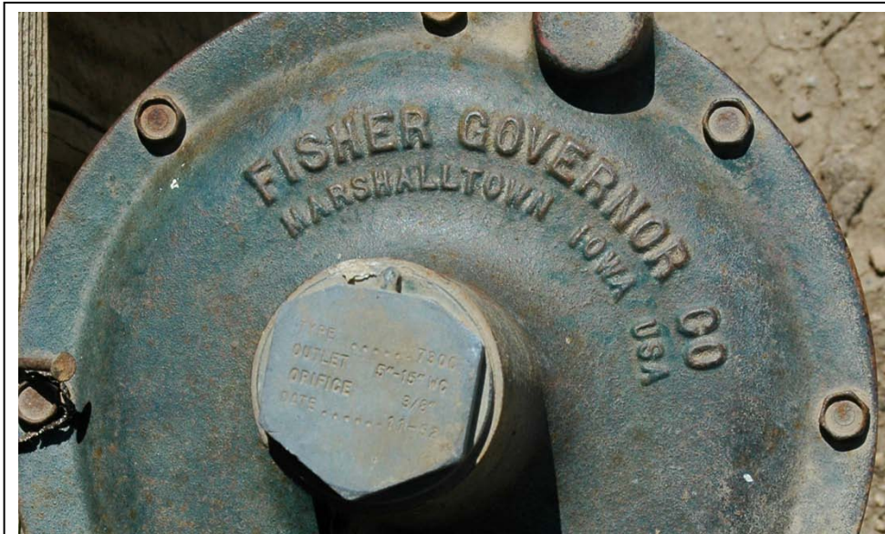
Figure 6.5: Gas valve installed on the exterior of Dorothy's House near the kitchen. Date reads 11/52.
