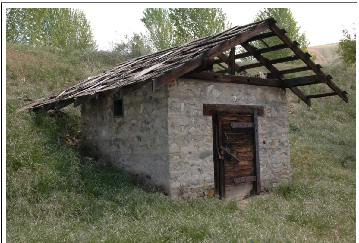
Figure 5.6: Cold storage shed built of native stone. May have been used at one point to store dynamite (Clendenen 2011). For its location within the complex of Headquarters, see Figure 5.5. See image 5.8 for detail above door.
