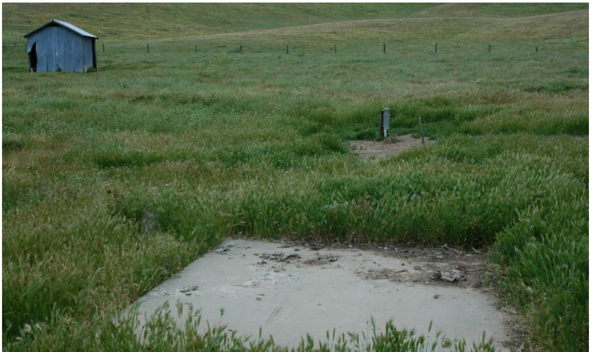
DSC_0296 – View toward the south. Foreground concrete platform, electrical power box with corrugated metal shed in the middle ground.
