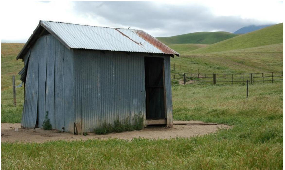
DSC_0279 – View toward southeast. Overview of corrugated metal shed. San Emigdio Hills in background.
