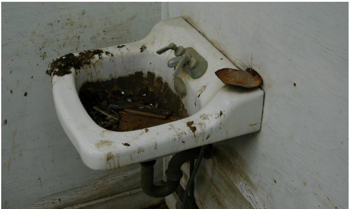
DSC_0329 – Bathroom sink and hardware. Note the re-use of tin can lid.
