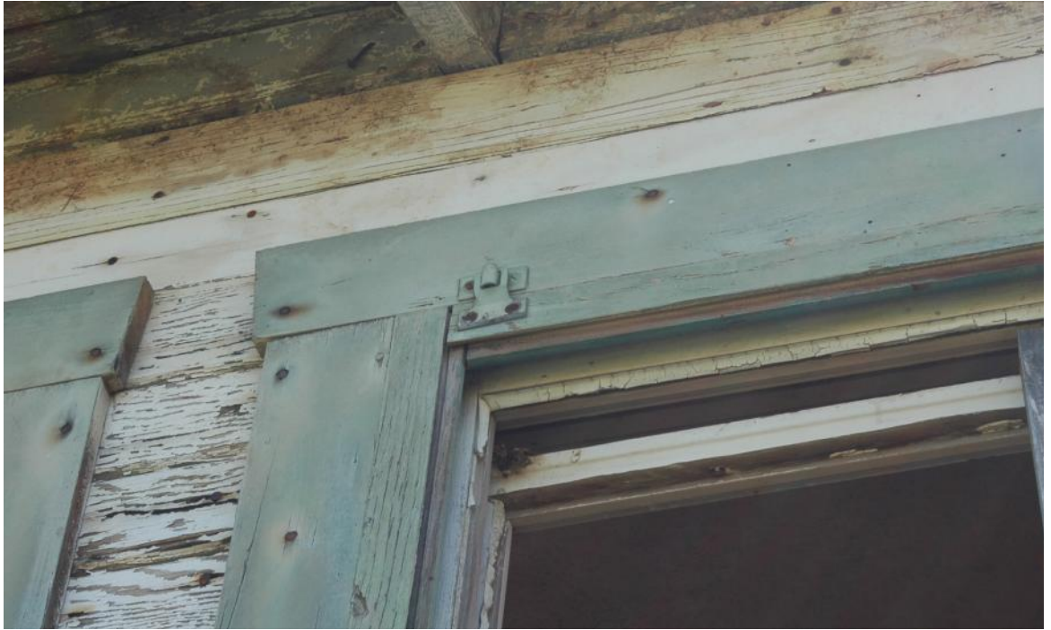
DSC_0430 – Enclosed north porch, exterior window hardware.
