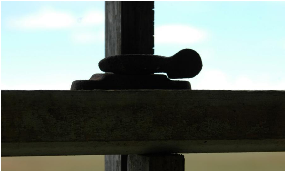
DSC_0343 – Window hardware on front porch windows.
