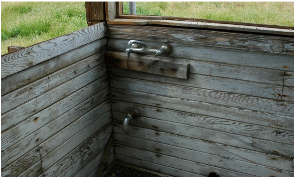
DSC_0315 – Sink hardware in the southern enclosed back porch.
