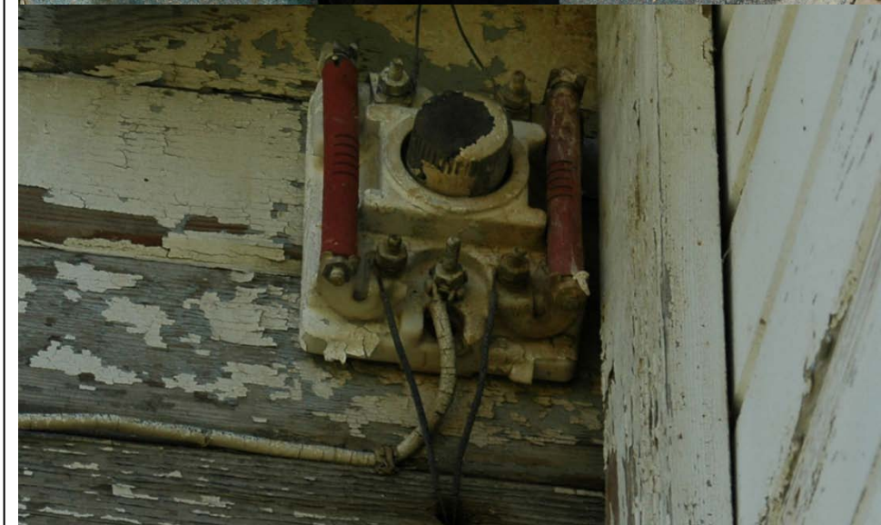
Figure 6.6: Electrical box installed on the exterior of Dorothy's House near the front porch.
