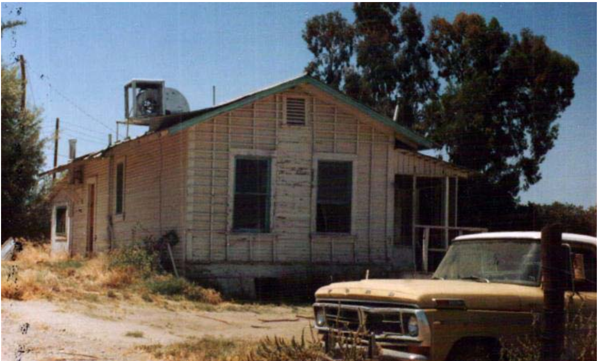
#68 – Looking West. House at San Emigdio.
