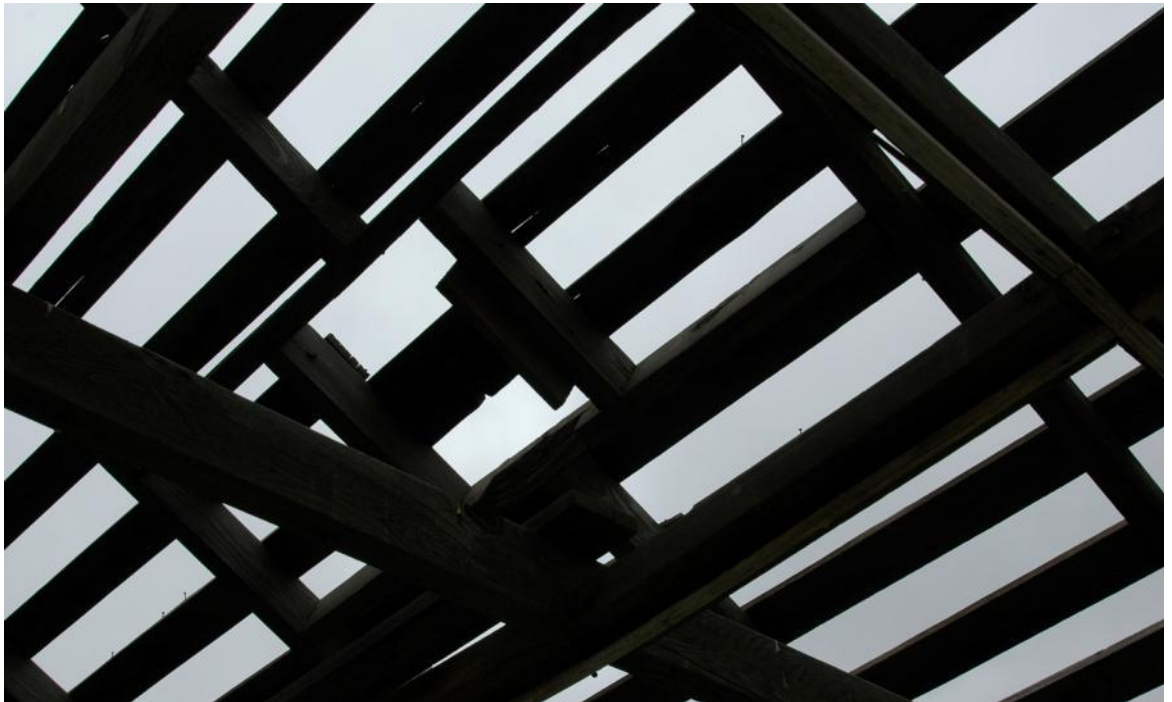
DSC_0351 – Rafters view over kitchen. Showing locale for stove exhaust.
