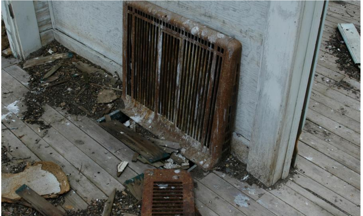
DSC_0325 – Central heating unit installed in central wall.
