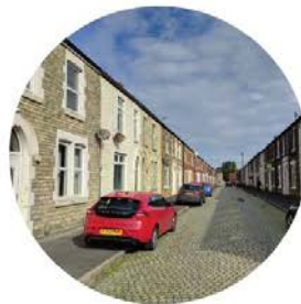
Victorian housing (repetition)
