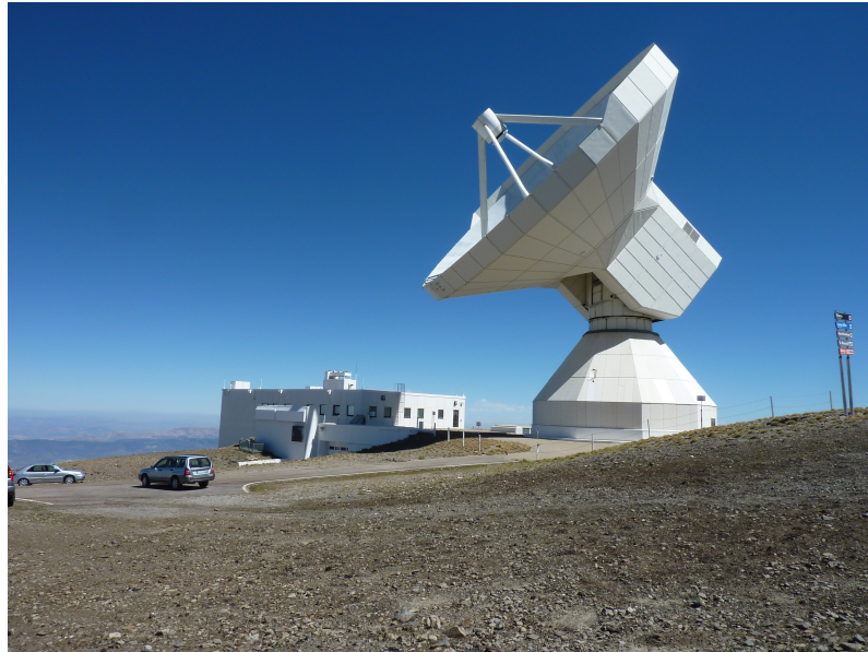
Figure 2.5: IRAM 30m telescope, showing the 30m dish, secondary reflector, mount and control room (credit: D. H. W. Glass).
