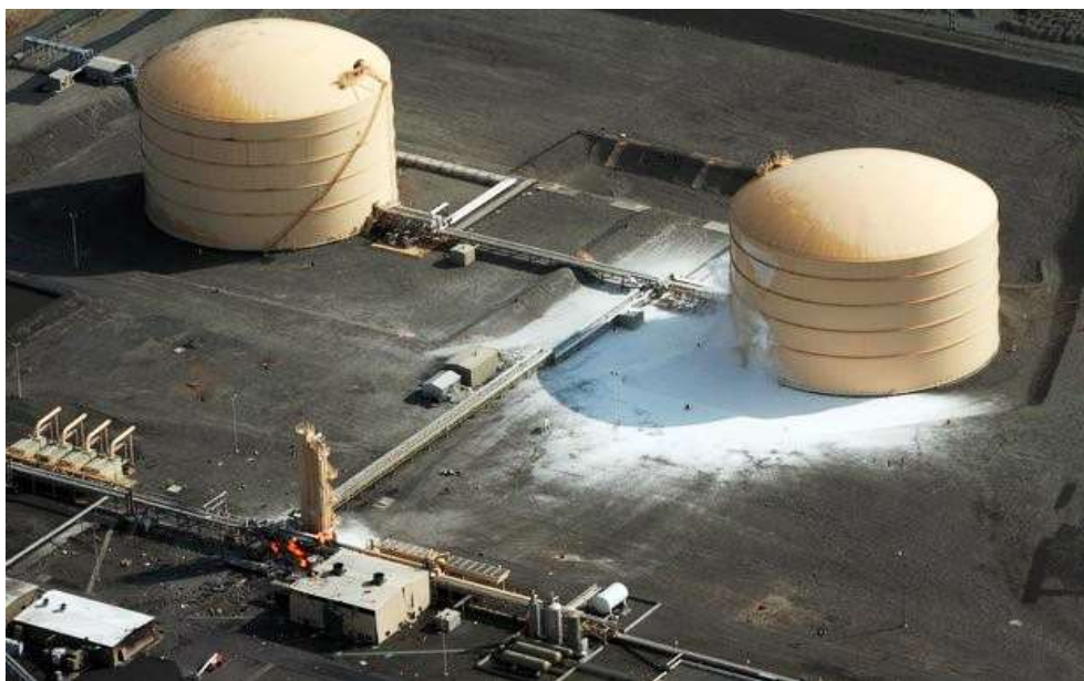
Figure 2.9: Tank explosion in LNG plant (Courtesy Wikipedia)
