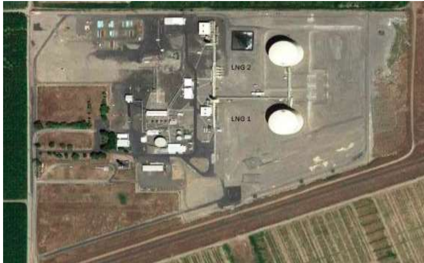
Figure 2.8: Aerial view of LNG Peak shaving plant (Courtesy google earth)
