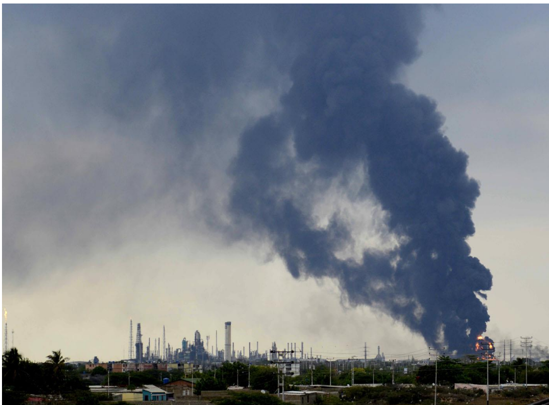
Figure 1.2: Final stage of Amuay Refinery fires, Venezuela [9].
