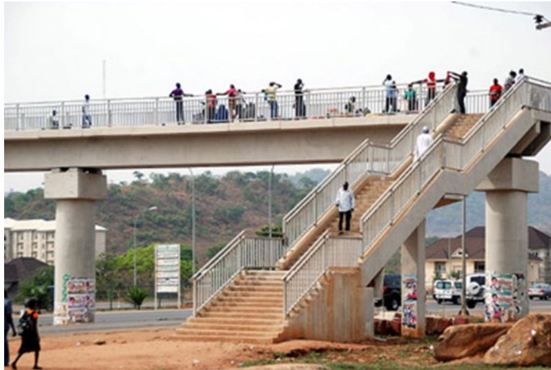
Picture 6: Pedestrian Bridge without Ramp
