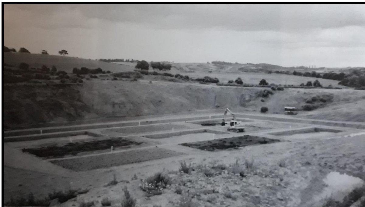
FIGURE 7.9 – Laying of subsoil treatments at Winterton in 1992. Manufacturing of subsoils was the first phase of ‘The Humberside Project: Making New Soils from Waste’. Organic amendment trials followed subsoil construction, and were a secondary phase of the Humberside project (Drobig, 1999; Hislop and Harding, 1999; Foot et al., 2003).
