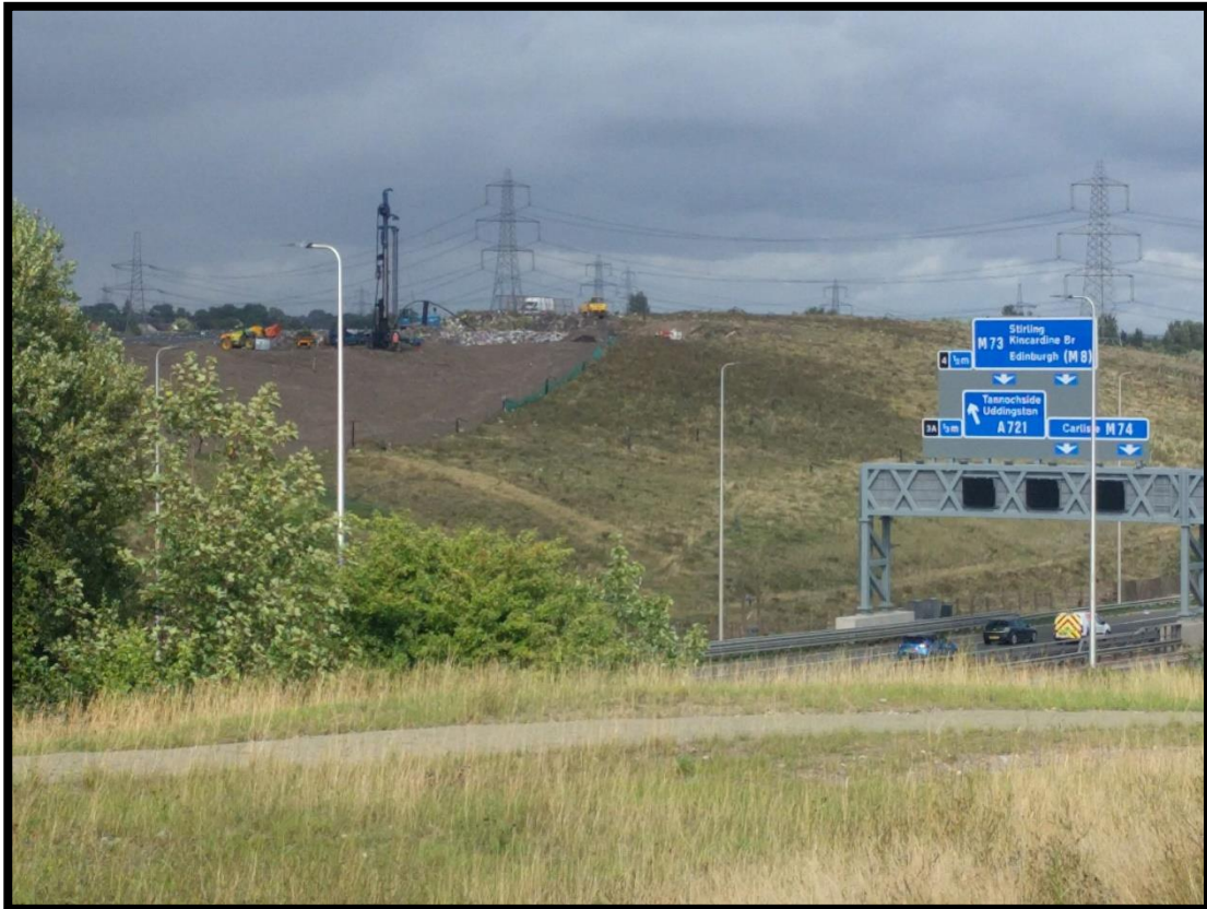
FIGURE 6.8 – Steep banks at GOH-SOUTH (foreground). The site overlooks the dividing M74, and GOH-NORTH landfill (background) where active areas of landfill can be seen.
