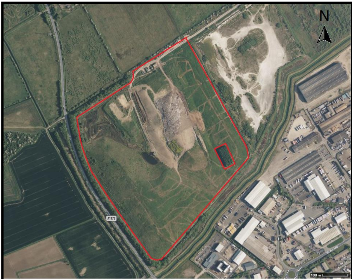
FIGURE 7.2 – Satellite image of Immingham landfill outlined in RED. The second of three near identical CGW related experiments was established here in 1997 (small RED square). The landfill receives non-hazardous waste and remains active at present. The large patch of white ground near the top of the image is the gypsum disposal bed.
