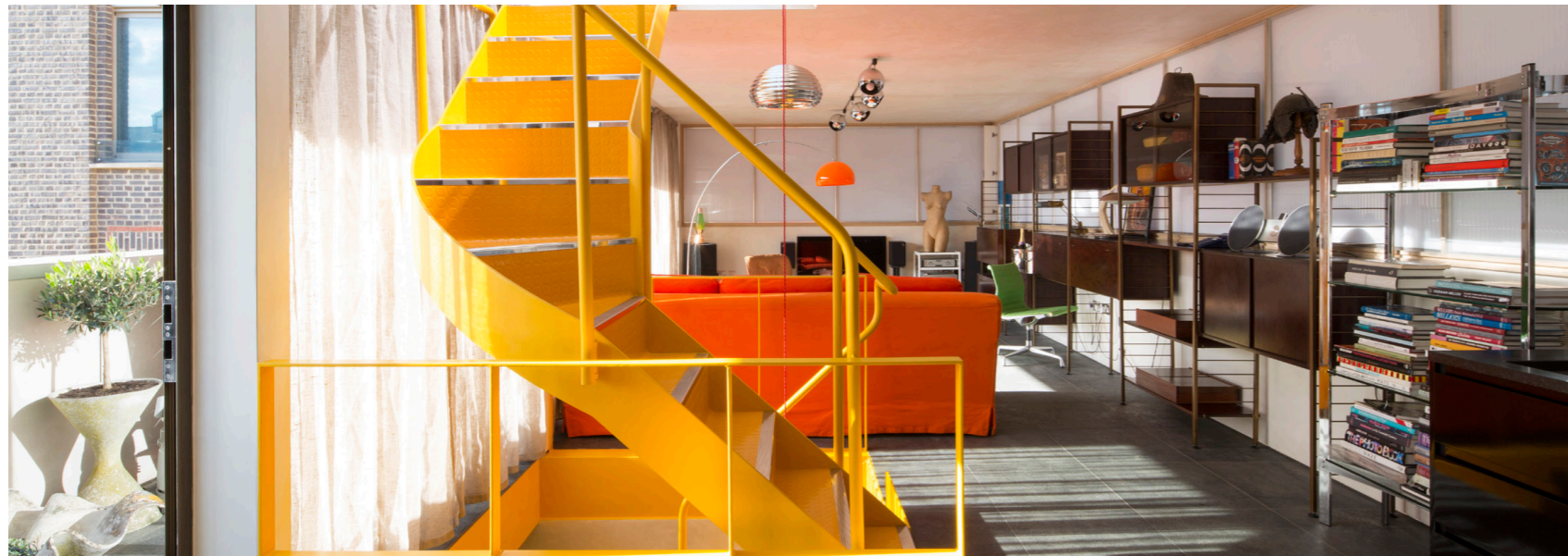
New 2nd Floor Helix Stair
