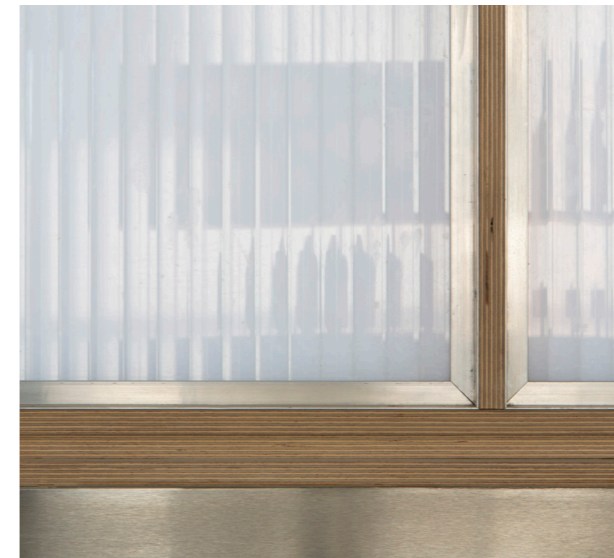
New lightweight translucent façade_Detail
