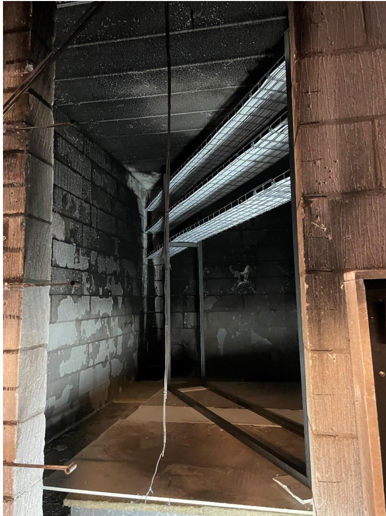
Figure 44: Picture of the final cable test set up in the ISO 9705 room.
