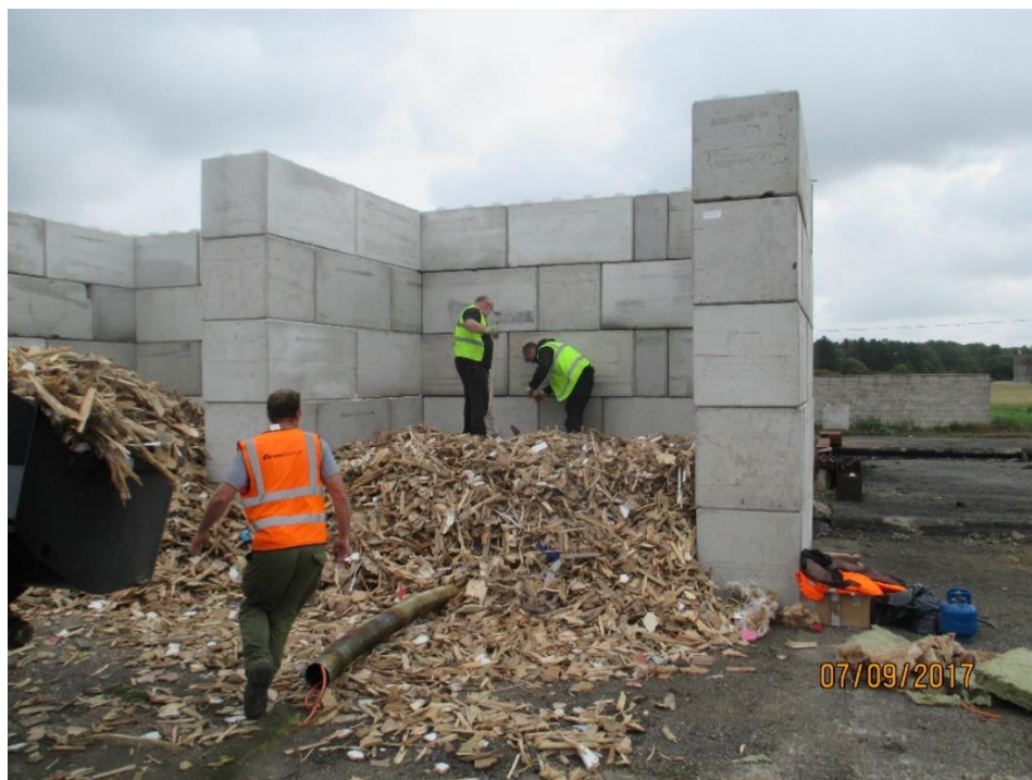
Figure 72: Test No 19 (table 2) thermocouple being positioned
