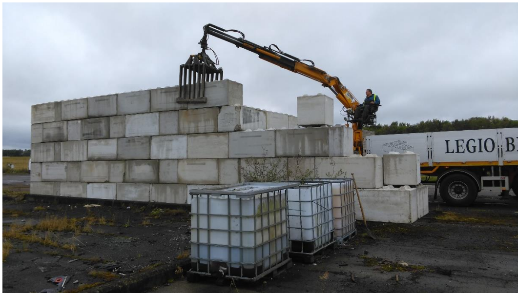
Figure 67: Legio block bunker under construction
