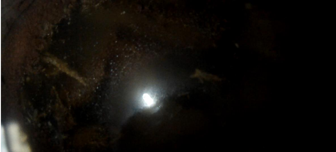
Figure 14: Underside of the test No2 15:30 PM condensation can be observed
