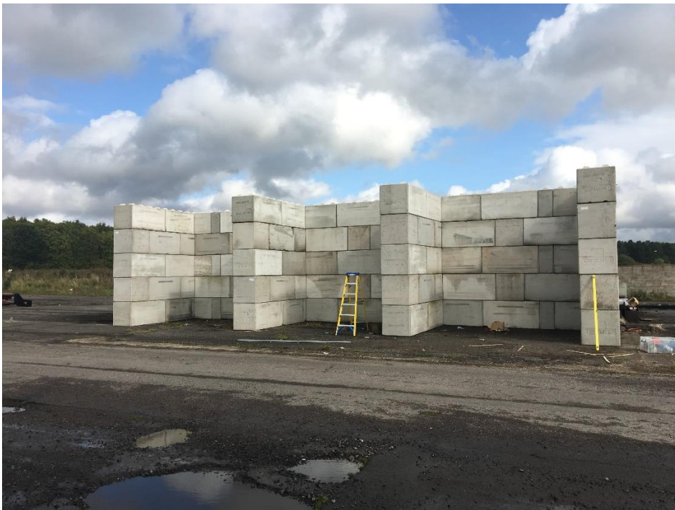
Figure 66: Concrete bunkers 5 m high and 3m by 3 m
