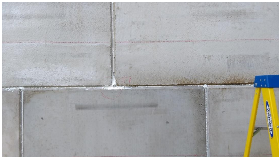
Figure 70: Test No 19 (table 2) gaps in the wall between the bays was sealed and thermocouple indicated by the red circle
