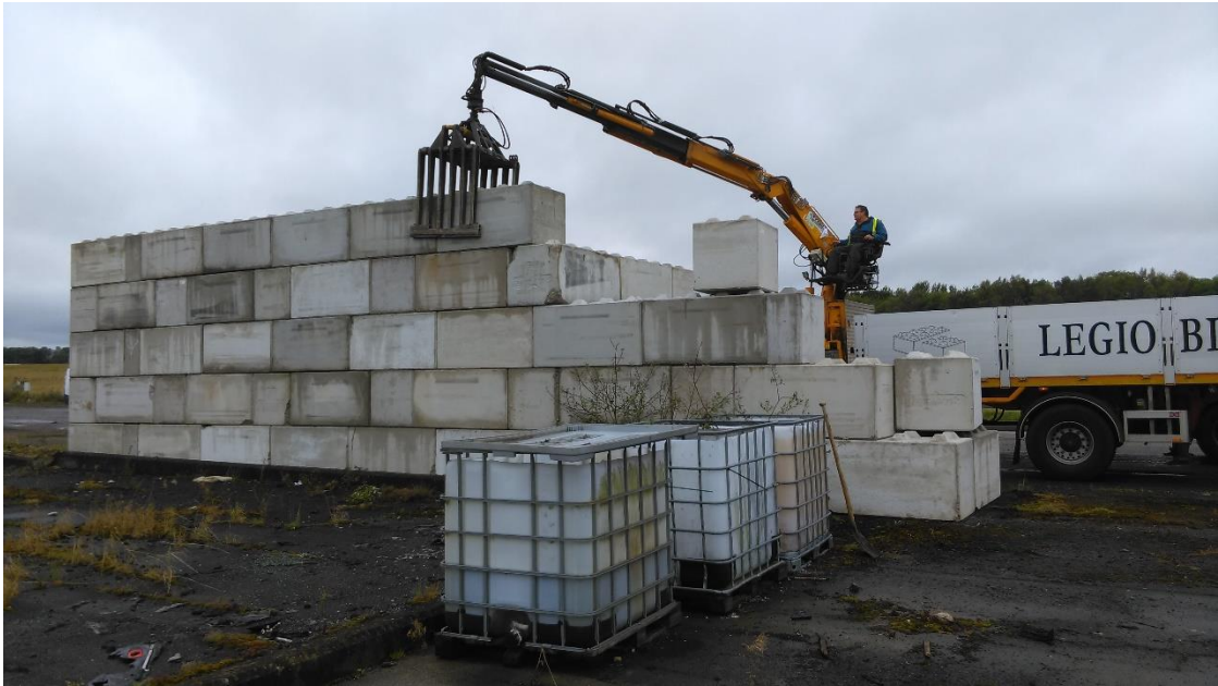
Figure 178: Legio wall being constructed
