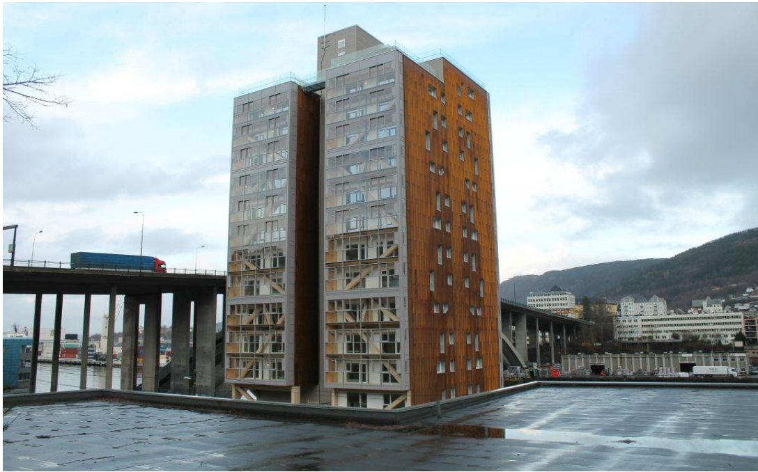
Figure 3. The Treet building, Bergen, Norway (Kjolberg, 2017)
