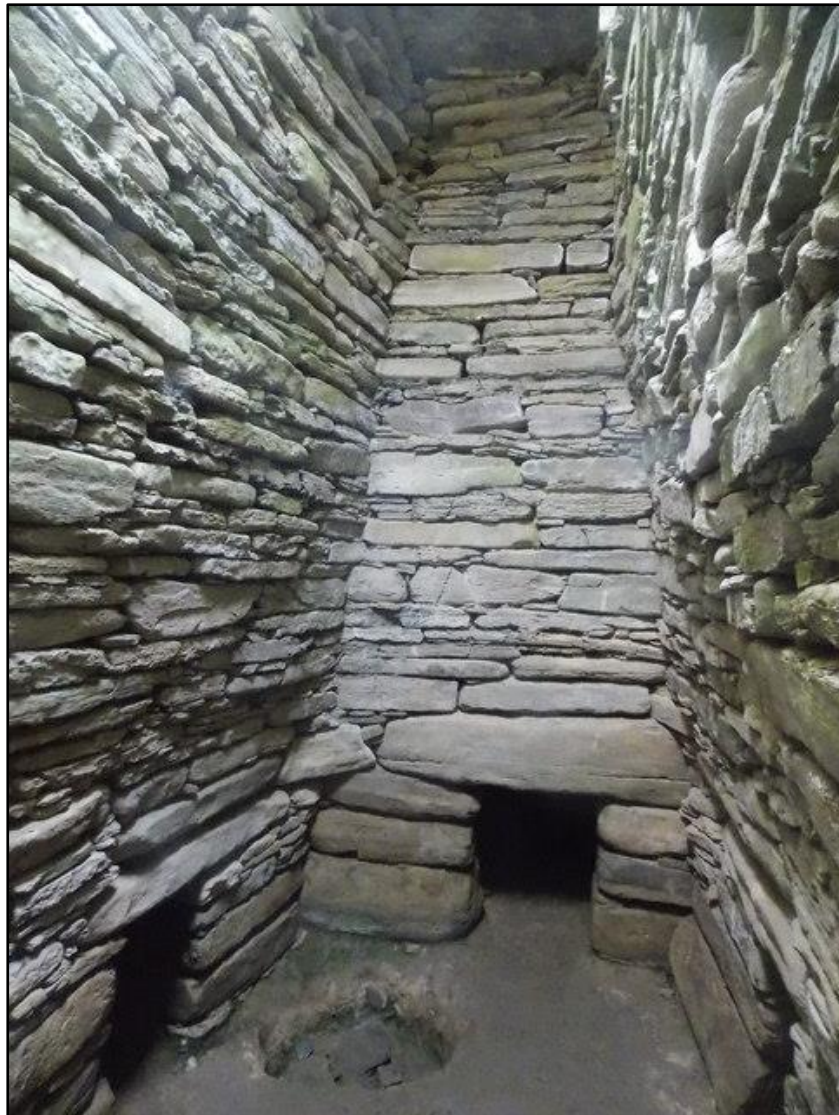
Figure 2.33. Dry stone corbelling effect within the chambered tomb as Quoyness, Sanday Orkney (authors own photograph 2021)
