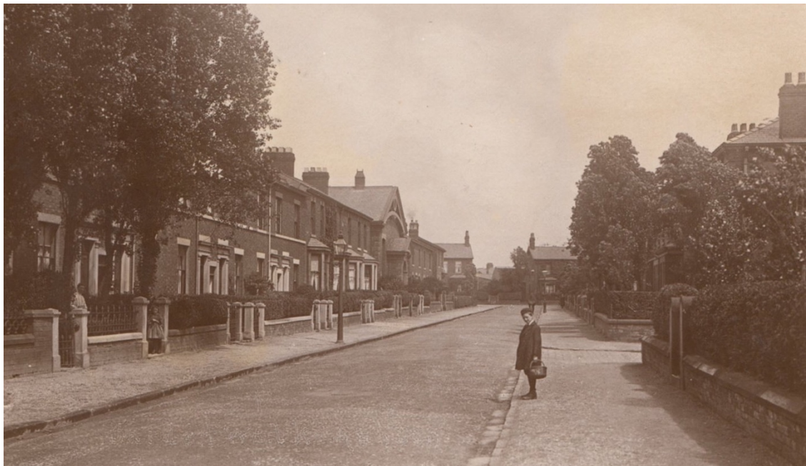
Fig 2.1 Garden Walk around 1900 showing Garden Walk Terrace on the left, with the later bay-fronted Ruby Terrace houses beyond.
