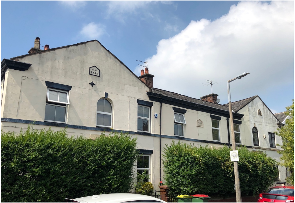
Fig 1.3 Spring Bank in 2020. Samuel Wilson's houses dated 1860, seen from Bank Place. Photographs from the 1970s show the brickwork unrendered.
