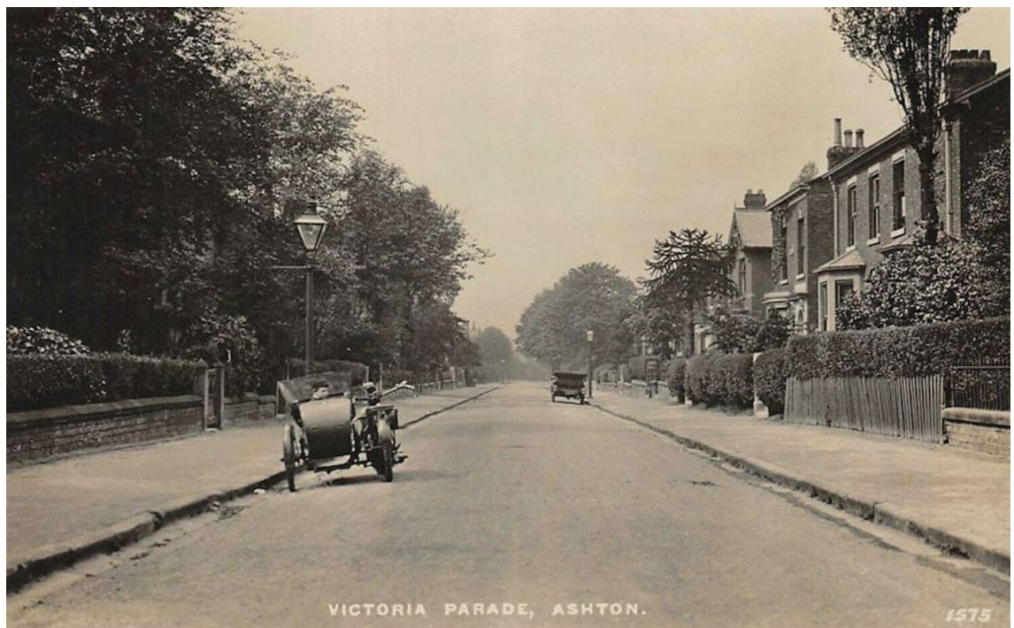
Fig 2.6 Victoria Parade in the 1920s. Sixty years after the creation of the estate, all plots are filled. The low walls and hedges required by the society are visible, but there is evidence on the right that some residents are disregarding the conditions. Preston Digital Archive
