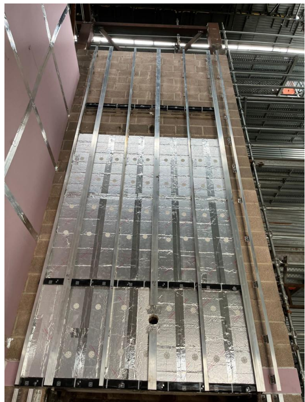
Test 2 - PIR insulation and mullions
