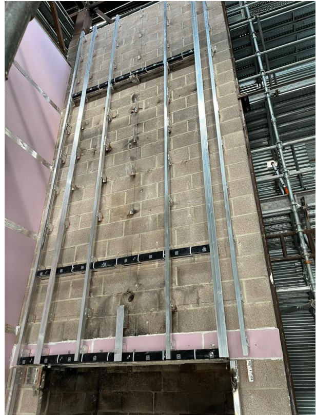
Test 2 - Horizontal cavity barriers
