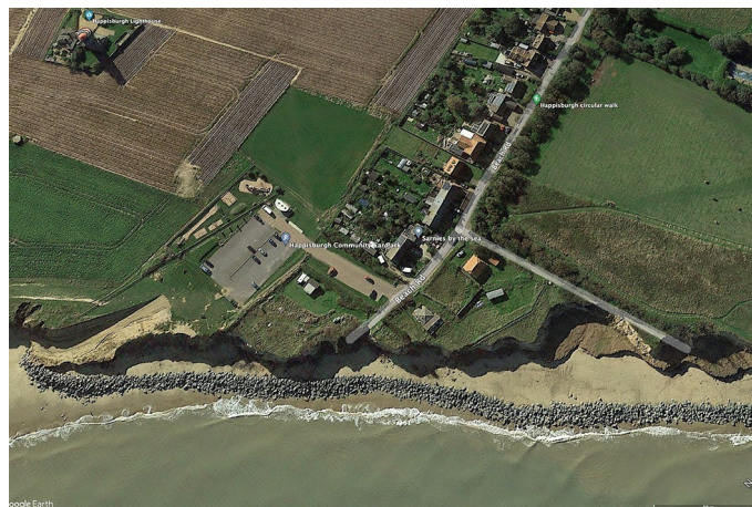
Fig. 4. Happisburgh coastal erosion in 2024. Source Google earth Pro maps, 2024.
