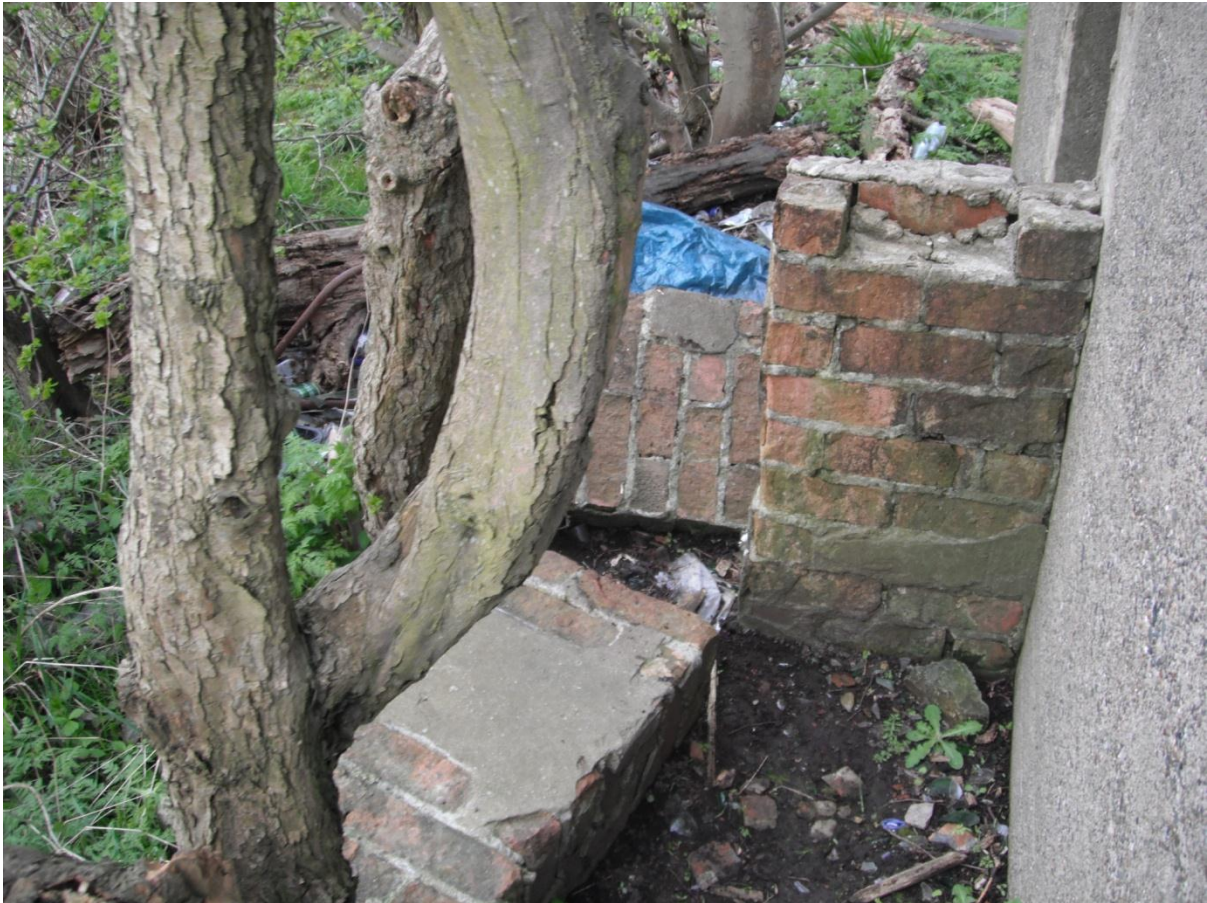
(Figure 4.18 Image of LA14 entrance sides, damaged and moved into a position to deny access to the pillboxes)
