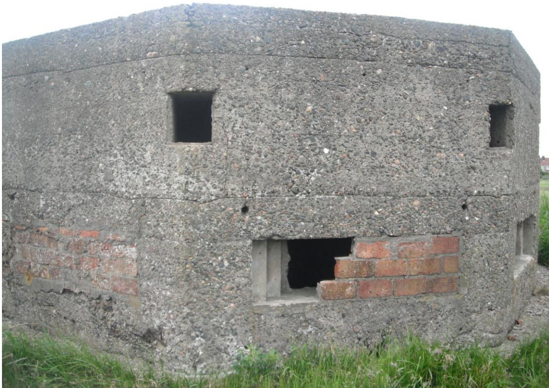
(Figure 5.3 Front section of CB10, showing alterations to the lower set of loopholes which had subsequently been altered via blocking)
