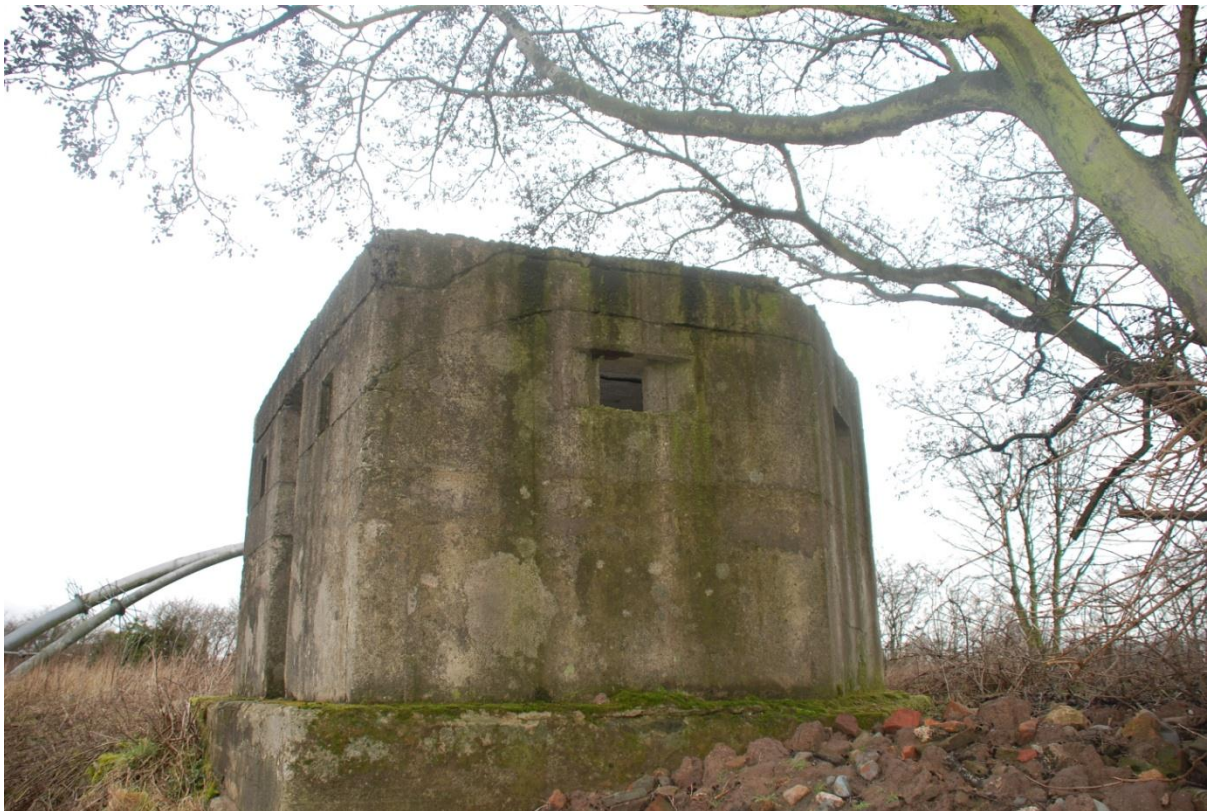
(Figure 4.16 Cracking above and below the loopholes LA02, with fracture lines along the entire pillbox)
