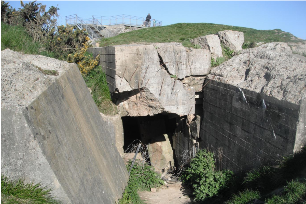
(Figure 4.21 Entrance to PH05 with heavy damage to the entrance roof and damage inside substantial so much that it has been blocked off with barbed wire)
