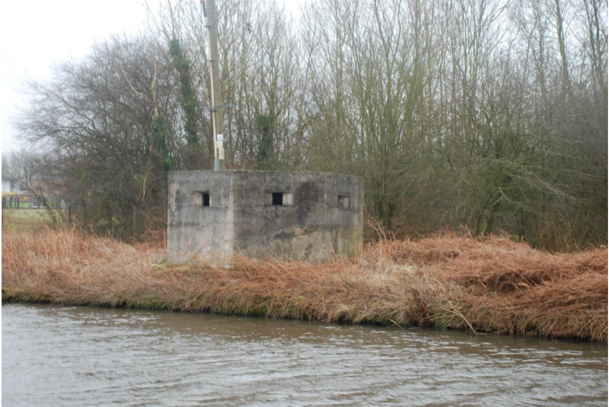
(Figure 1.1 LA01 adjacent to the south bank of the Leeds-Liverpool Canal. A FW3/Type 24 design, it is considered a common type of pillbox found in Britain)
