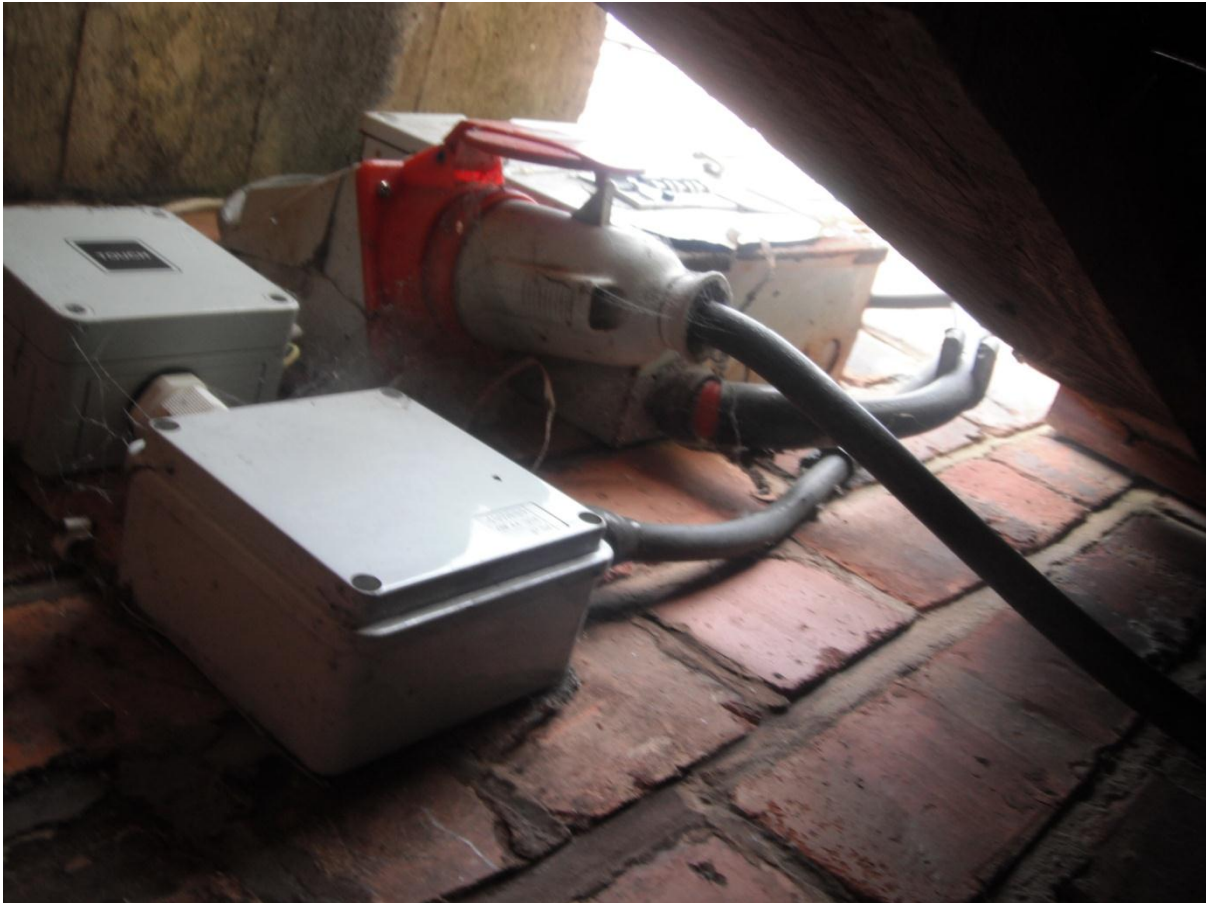
(Figure 4.24 Lower section of LA07. At the entrance electrical service boxes for the floodlight has been attached on the second floor)
