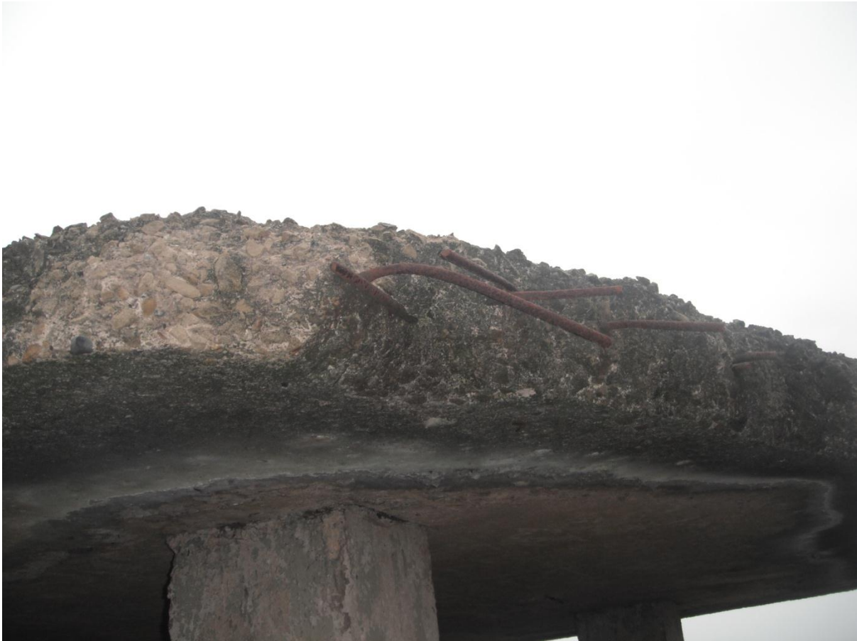
(Figure 4.17 Damage on the South-East corner of LA10)
