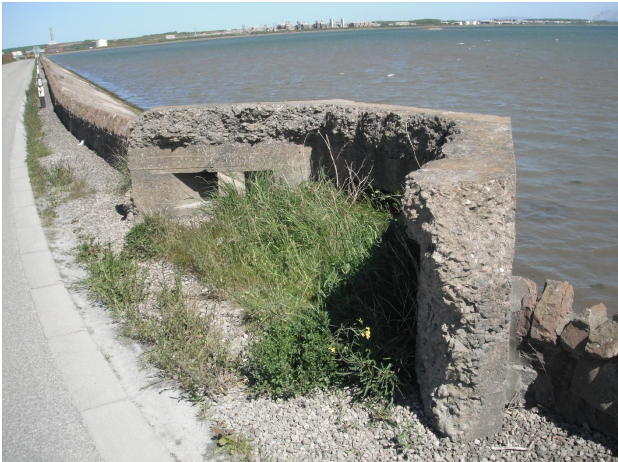
(Figure 4.19 Showing what remains of CB06, and the substantial weathering along the edges of the structure)
