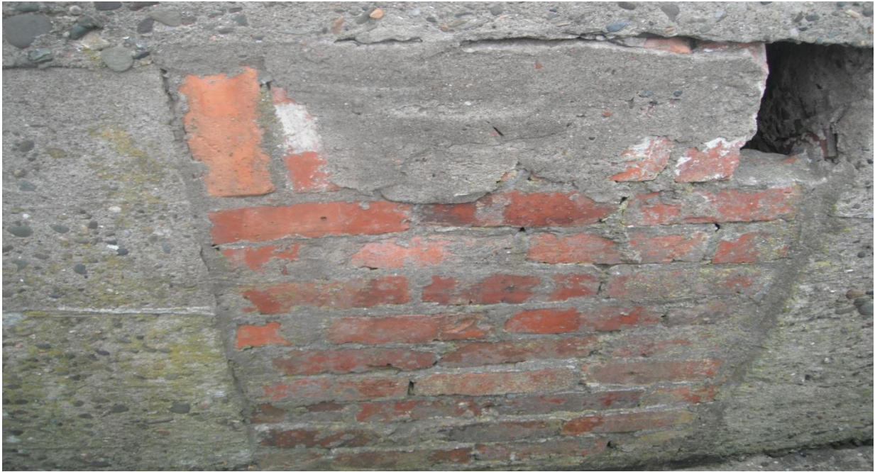
(Figure 4.11 Entrance to CB10 that has been completely blocked up using concrete and bricks)
