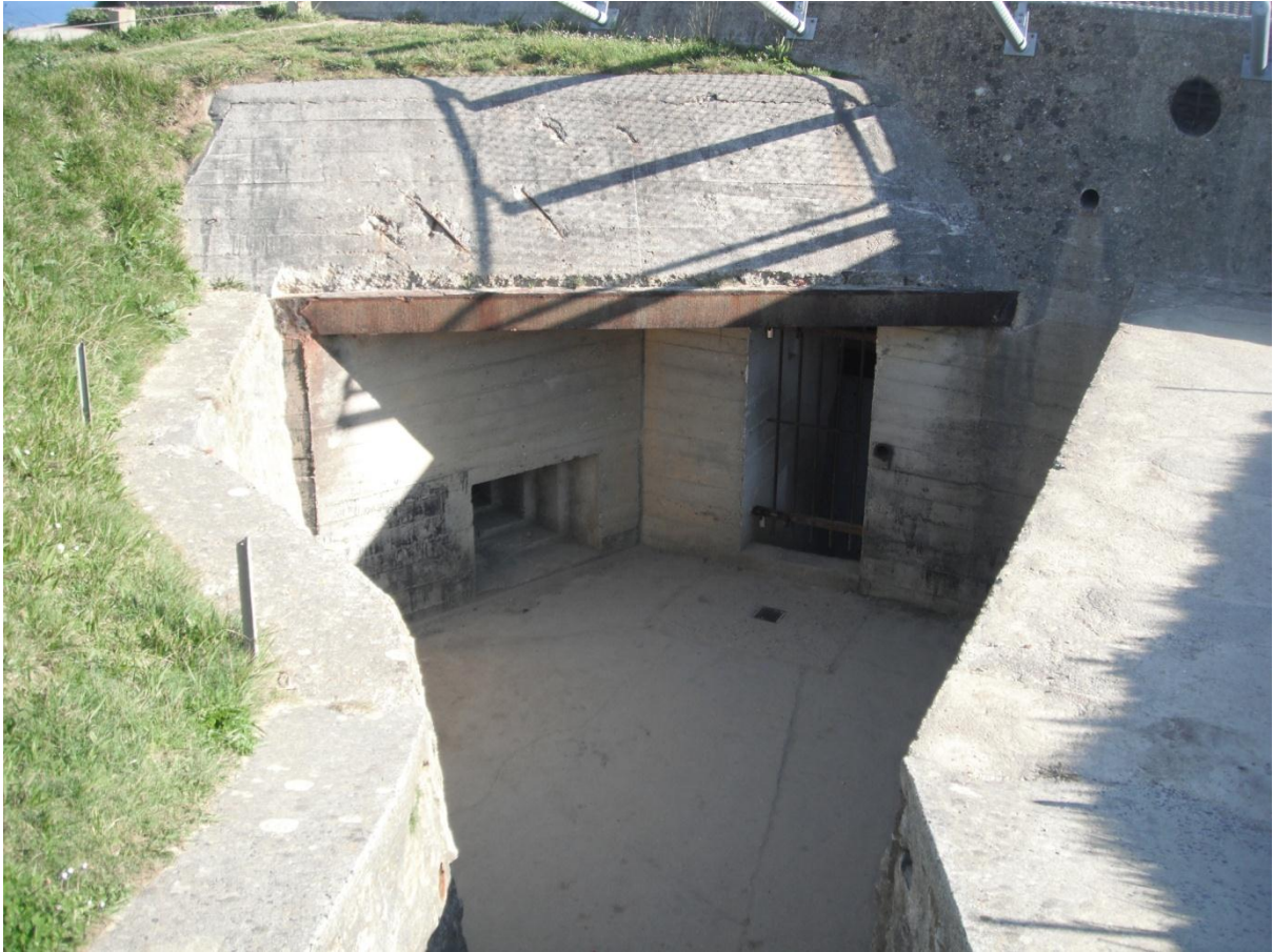
(Figure 4.31 Entrance to the observation bunker at PH09. The entrance has been gated for safety reasons)
