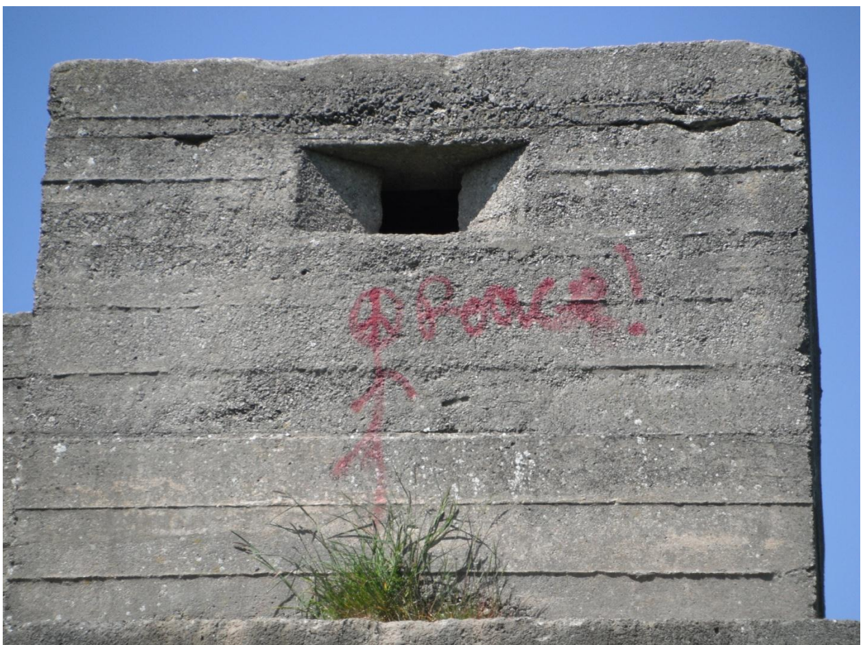
(Figure 5.7 Front exterior wall of CB05, with graffiti painted onto the surface,
