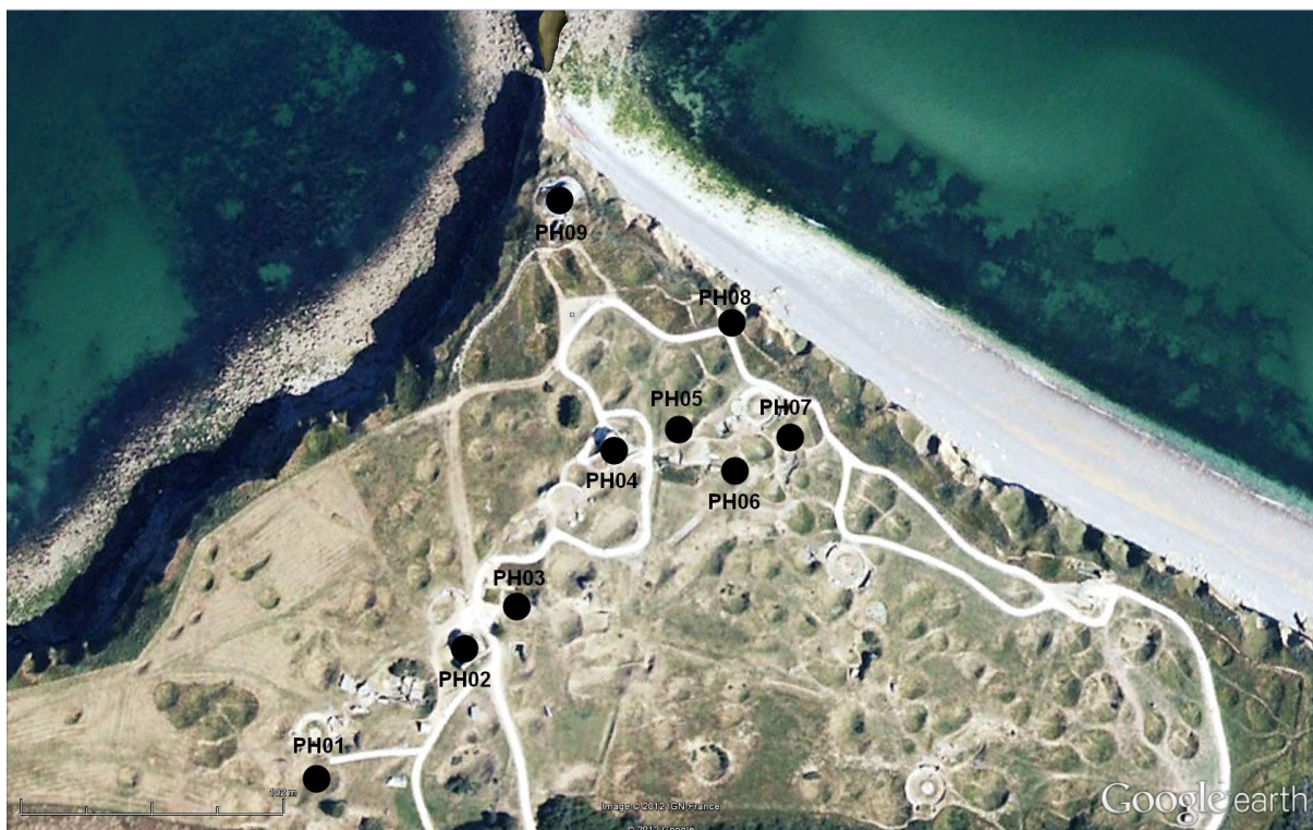
(Figure 4.10 Overview of the location of defensive structures at Pointe du Hoc)
