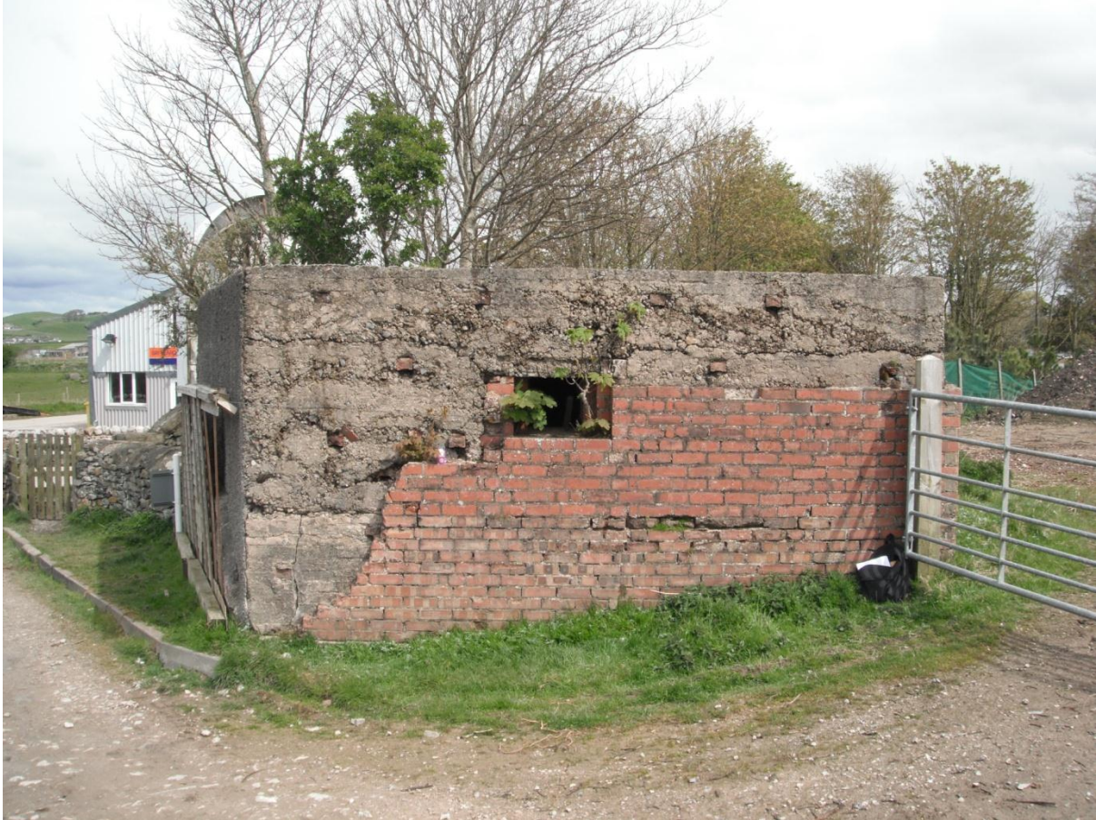
(Figure 4.29 CB14 located next to Lakeland Leisure Park, an unknown design with only one loophole)
