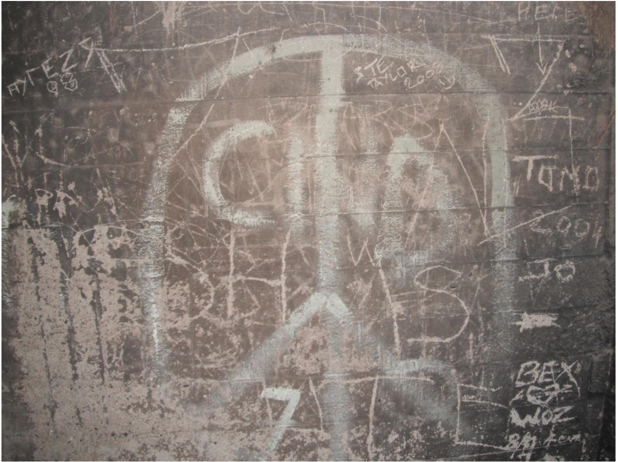
(Figure 5.9 Wall B of pillbox CB08 with layers of graffiti from various points in time)
