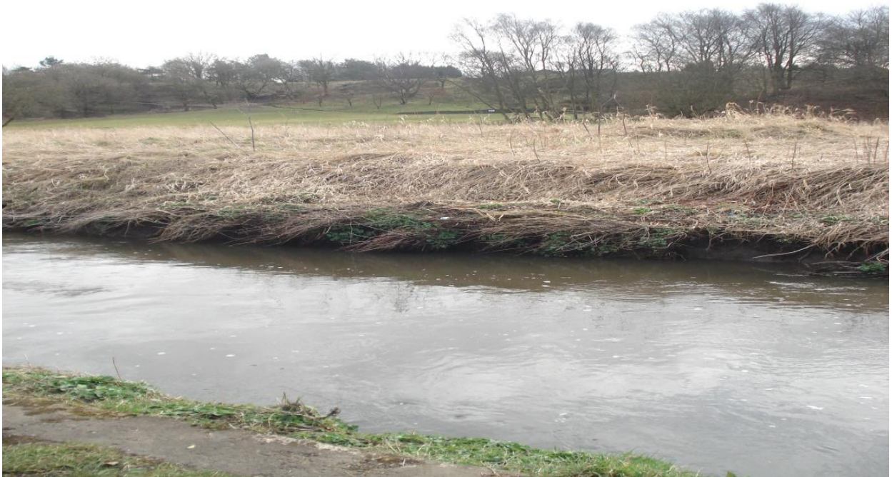
Fig. (13): Location 5, Ground View.
