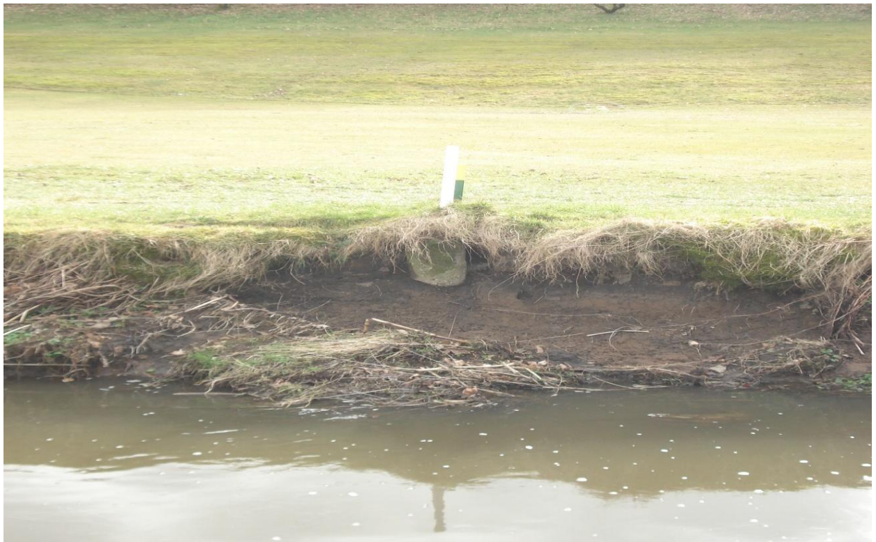
Fig. (9): The South bank, approximately 30 yards to the west of location 3, shows evidence of erosion and sand superficial deposits.
