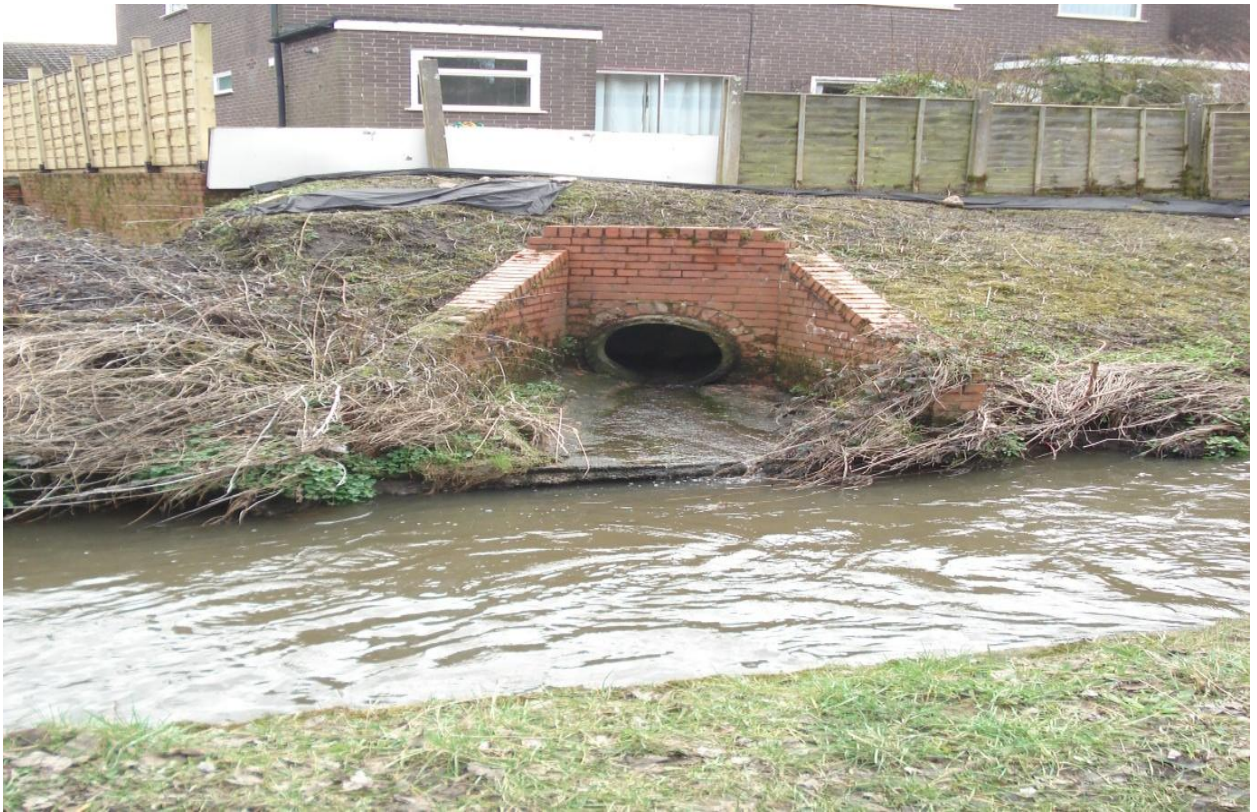
Fig. (4): Surface water discharge from the housing estate, between Locations 1 & 2.
