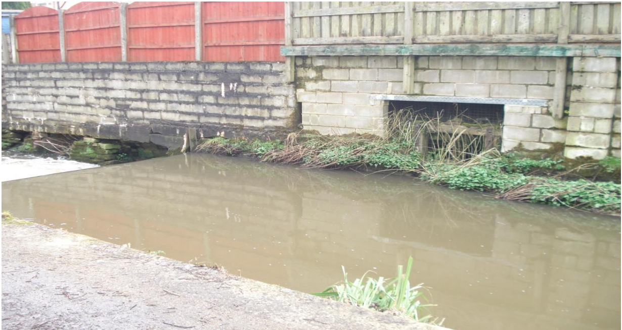
Fig. (2): Location 1, Ground view.
