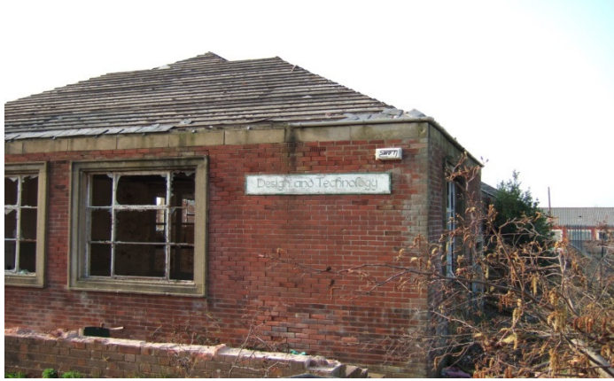
Figure 5 Destruction of the Design and Technology building.
