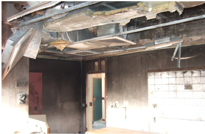
Wires hanging from the ceiling (Jackson, 2012).
