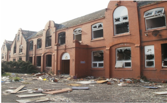
Figure 8 Decay and dereliction of Fylde Farm School (front of the school).
