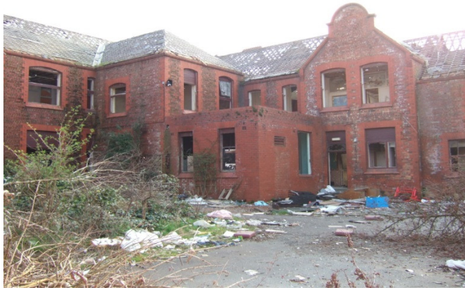
Figure 6 Decay and dereliction of Fylde Farm School (rear of the school).
