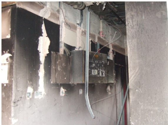
Wires hanging out of the wall (Jackson, 2012).
