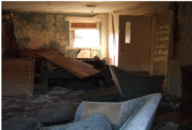
Complete destruction and vandalism (1) (Jackson, 2012)
