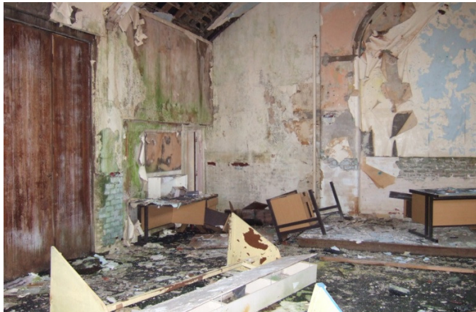
Complete destruction and vandalism (2) (Jackson, 2012)
